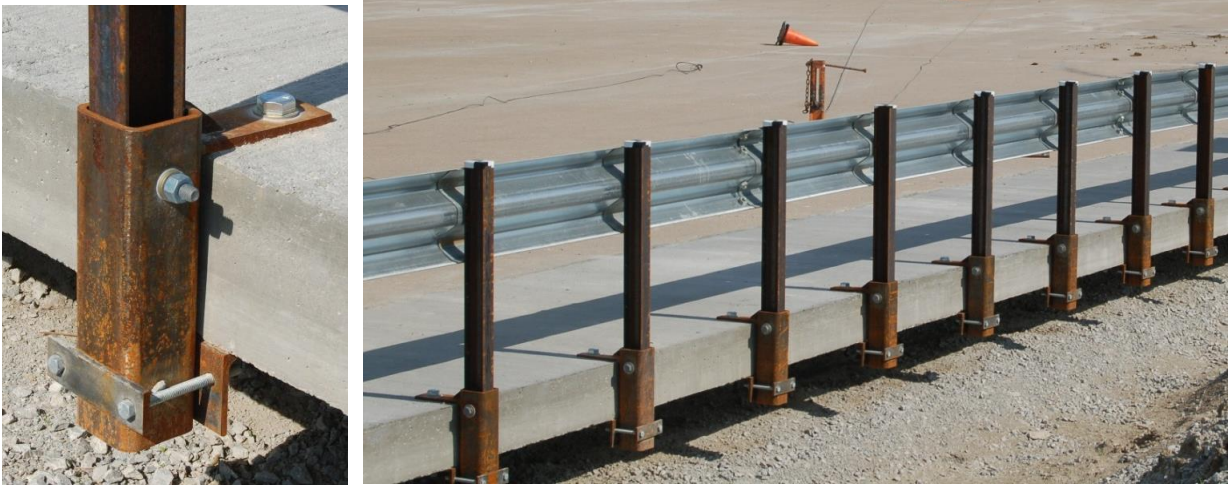
Figure 2. MGS Bridge Rail Installation
