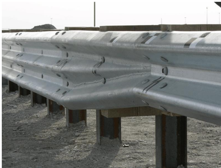
Figure 19. MGS Stiffness Transition with Asymmetrical Element [21]
