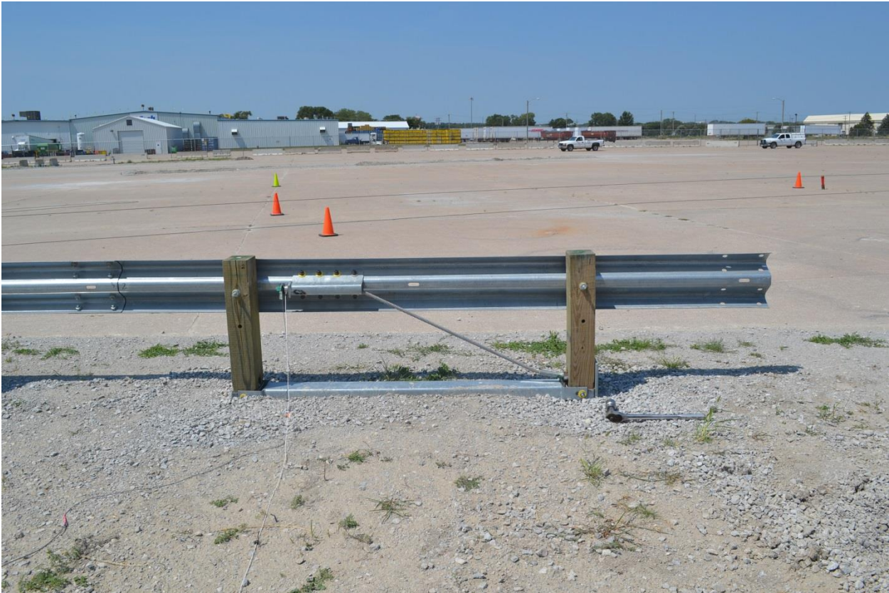
Figure 18. Load Cell Placement, Test No. MGSS-1
