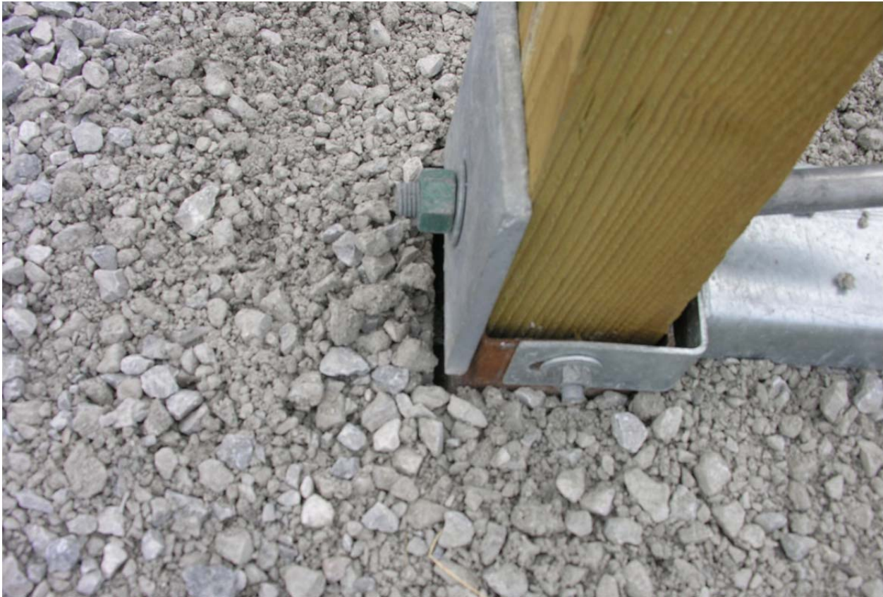
Figure 63. Soil Gap at Upstream End Anchor, Test No. MGSMRH-2
