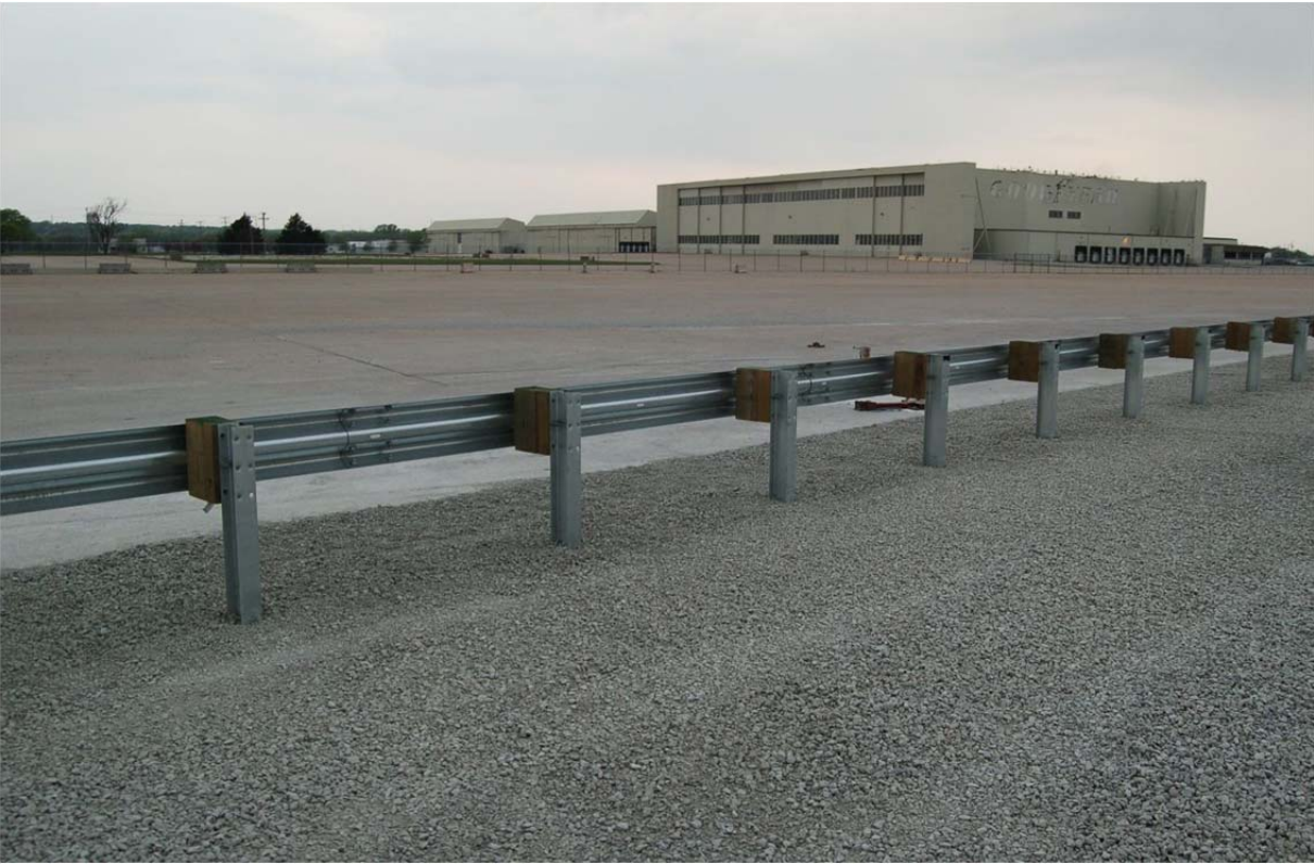
Figure 28. Test Installation Photographs, Test No. MGSMRH-1
