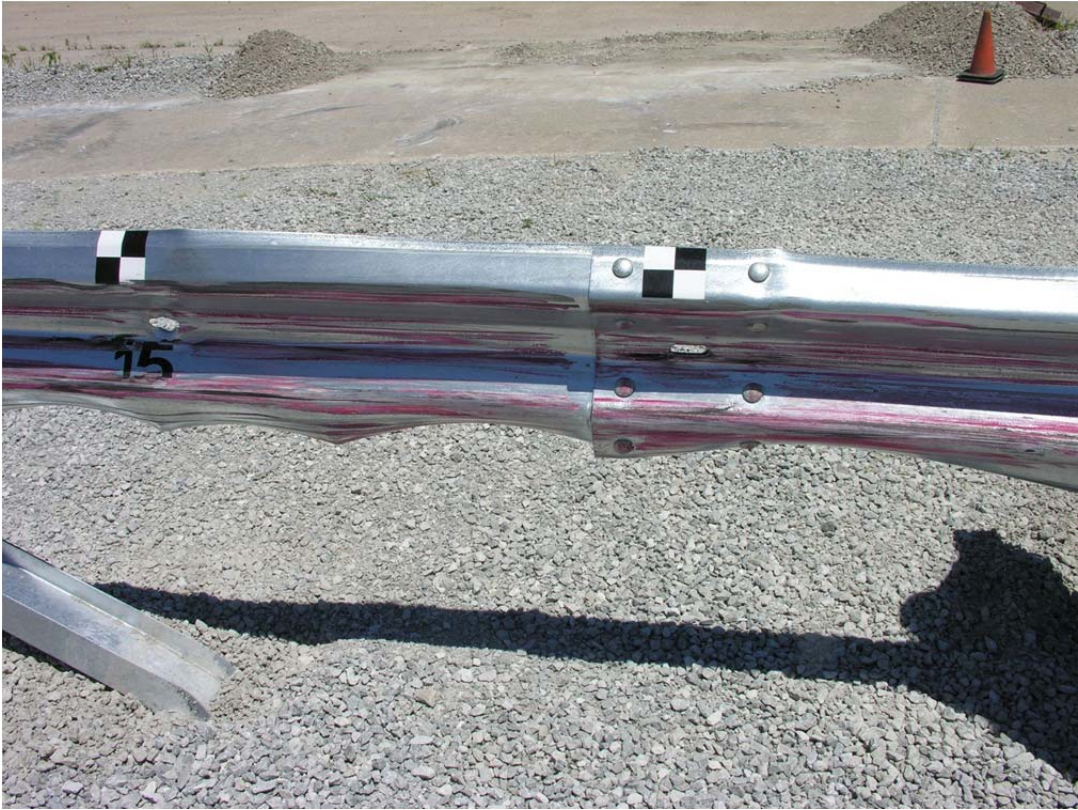
Figure 39. System Damage, Test No. MGSMRH-1
