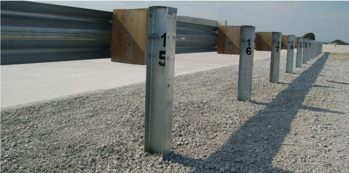
Figure 53. Test Installation Photographs, Test No. MGSMRH-2
