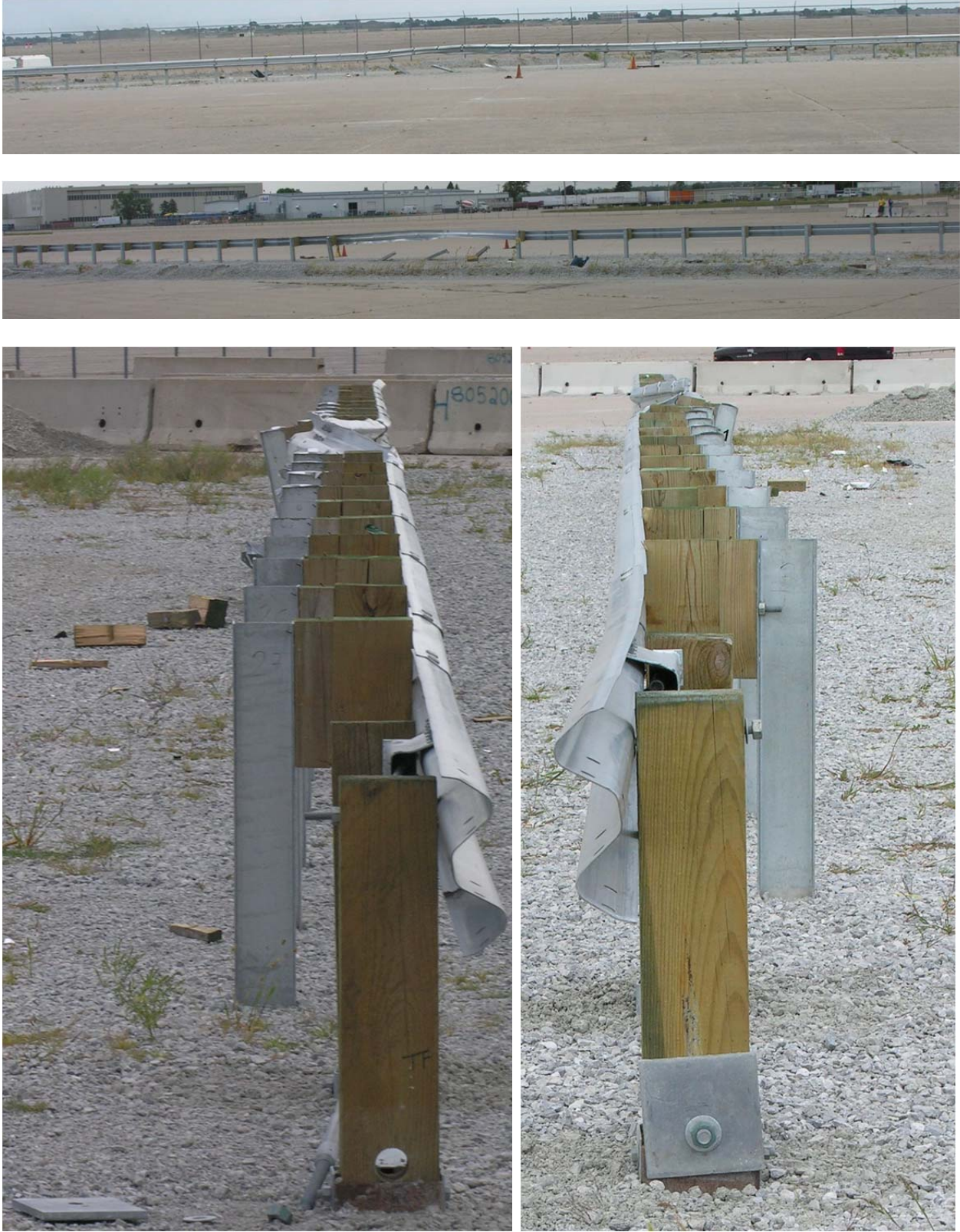
Figure 61. System Damage, Test No. MGSMRH-2
