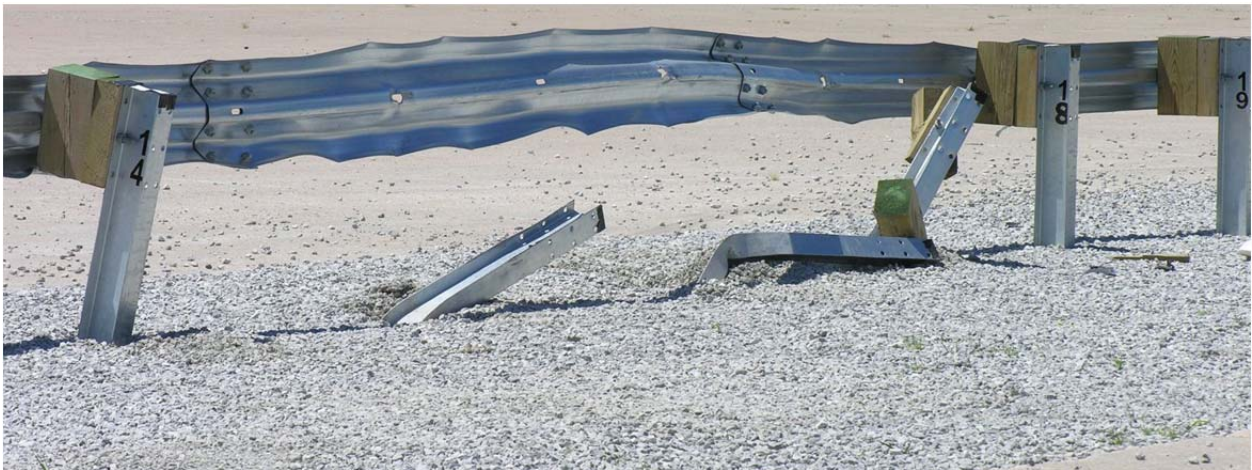
Figure 38. System Damage, Test No. MGSMRH-1
