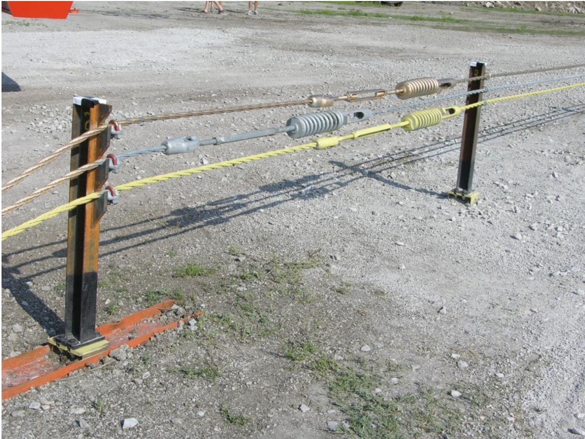
Figure 4. Generic Low-Tension Cable End Terminal
