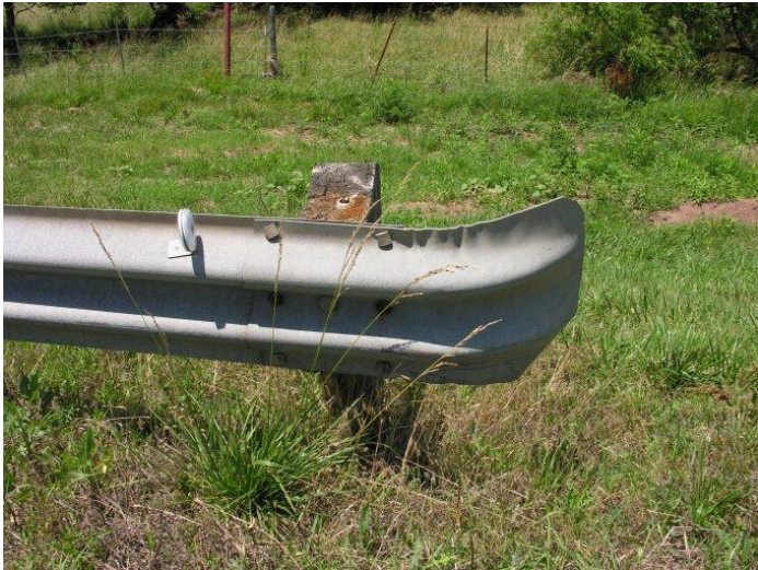
Figure 12. Examples of Existing W-Beam Guardrail Systems
