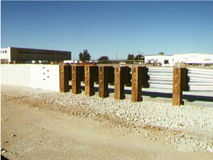
Figure 2. Generic W-Beam-to-Thrie Beam-to-Concrete Bridge Rail Transition
