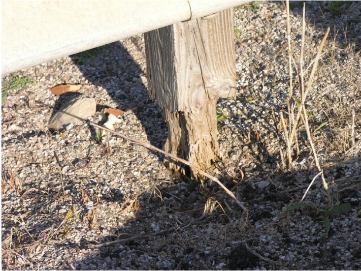
Figure 18. Examples of Missing and Inadequate Posts
