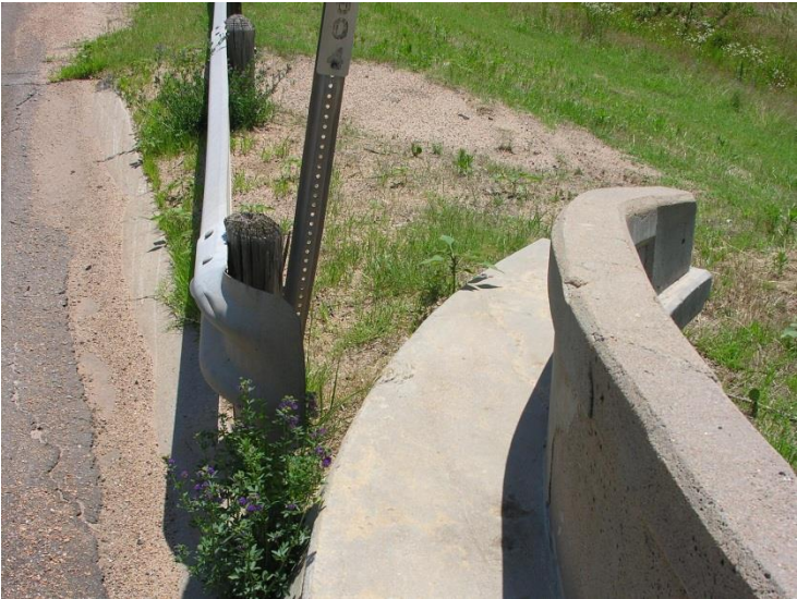
Figure 16. Examples of Existing W-beam Guardrail to Bridge Rail Transitions
