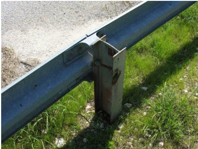
Figure 25. Examples of Channel Rail Systems
