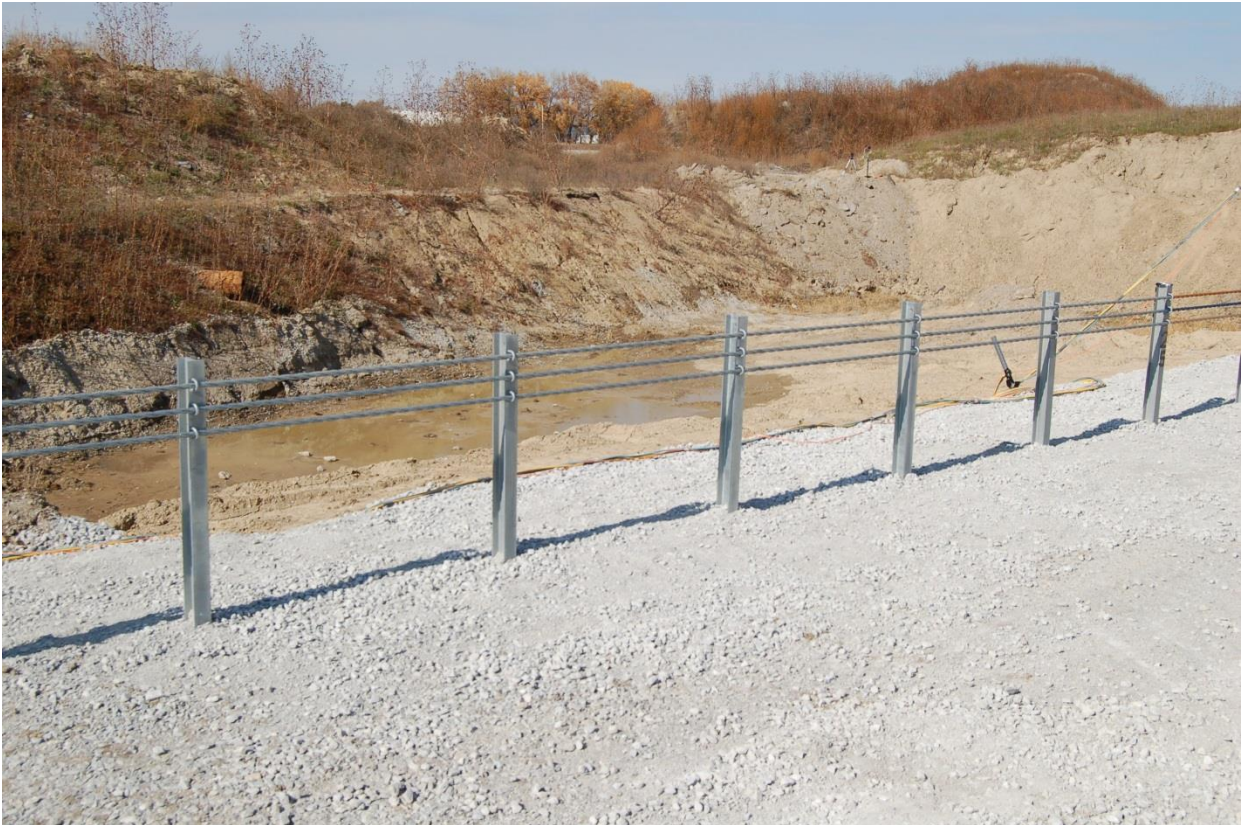
Figure 3. Generic Three-Cable Low-Tension Barrier
