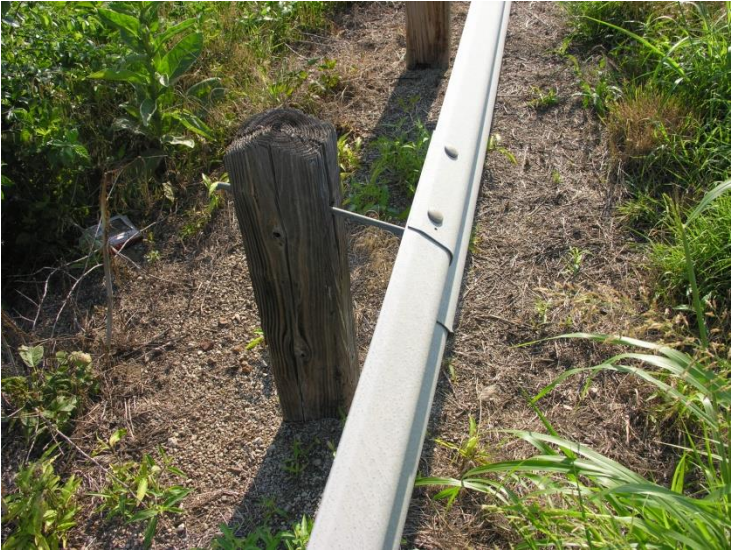
Figure 20. Examples Missing Blockouts in Existing Systems
