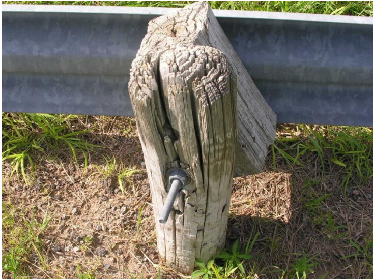
Figure 19. Examples Weathered and Decaying Post in Existing Guardrail Systems
