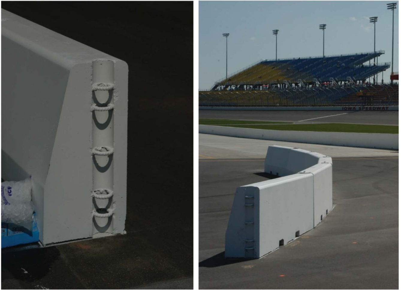
Fig. 1. Temporary concrete barrier design for Iowa Speedway.
