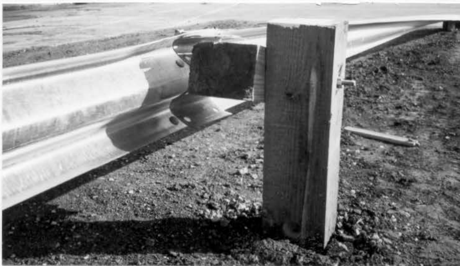
FIGURE 21. Damage at Post No. 1, Test NETD-1
