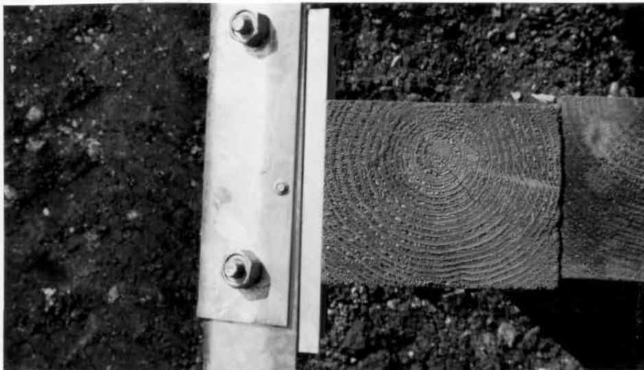
FIGURE 6. Guardrail Connection Detail, Post No. 3
