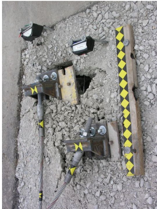
Figure 38. Anchorage Displacement, Test No. TTCB-1
