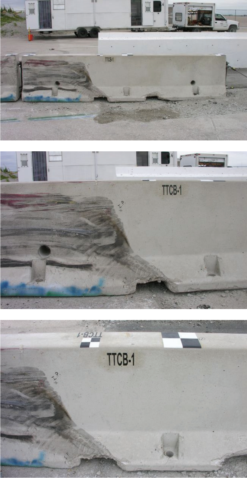
Figure 34. System Damage - Barrier No. 1, Test No. TTCB-1
