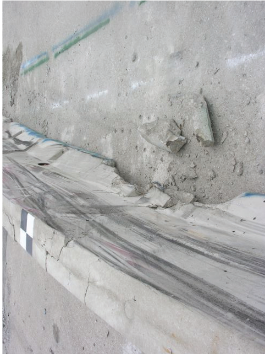
Figure 35. System Damage - Barrier No. 2, Test No. TTCB-1
