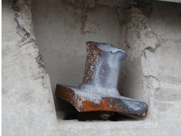
Barrier No. 1 Traffic Side Downstream
