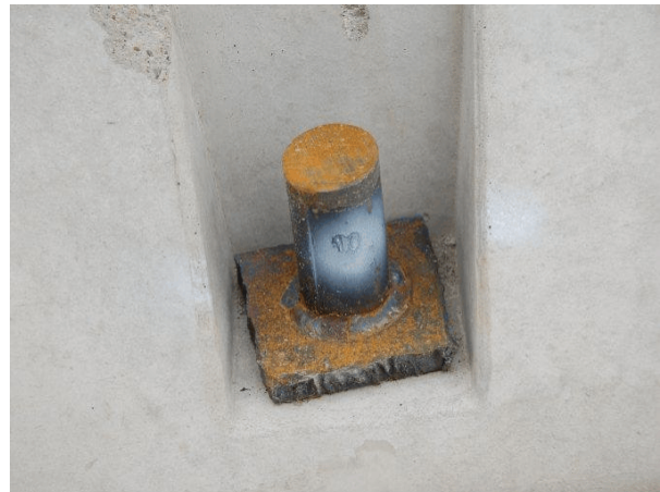
Barrier No. 2 Non-Traffic Side Downstream
