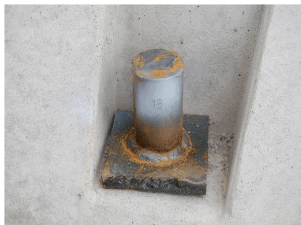
Barrier No. 4 Non-Traffic Side Downstream
