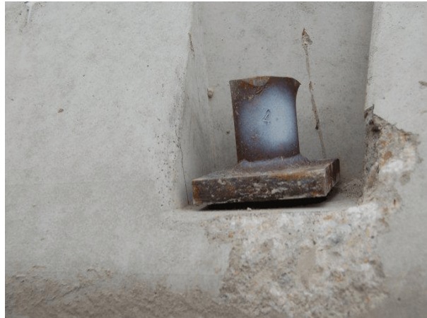
Barrier No. 1 Non-Traffic Side Downstream
