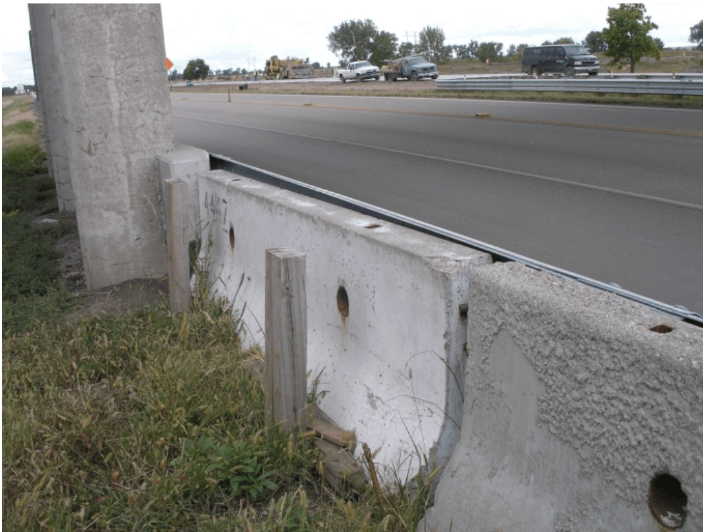
Figure B-8. Nebraska Temporary Barrier Transitions
