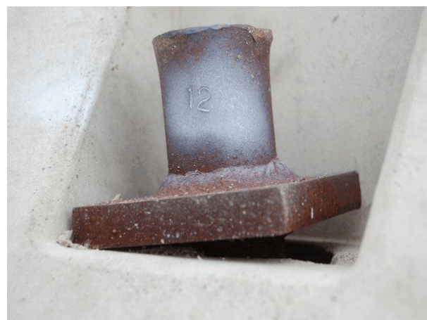
Barrier No. 2 Non-Traffic Side Upstream
