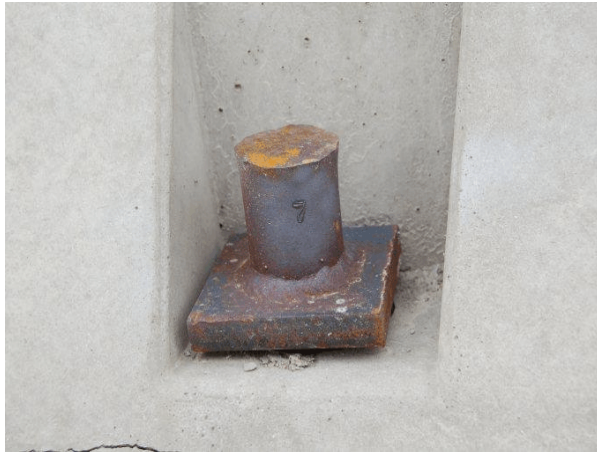
Barrier No. 2 Traffic Side Downstream
