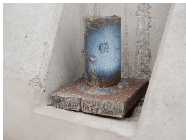
Barrier No. 2 Non-Traffic Side Midspan
