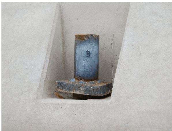
Barrier No. 2 Traffic Side Midspan
