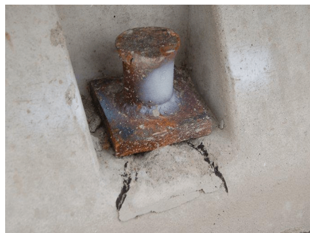
Barrier No. 1 Non-Traffic Side Upstream
