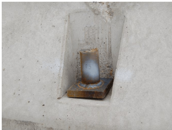
Barrier No. 3 Non-Traffic Side Downstream
