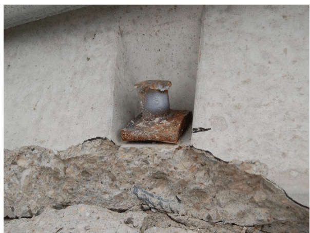
Barrier No. 1 Non-Traffic Side Midspan
