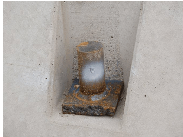
Barrier No. 3 Non-Traffic Side Upstream
