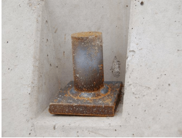
Barrier No. 3 Traffic Side Downstream
