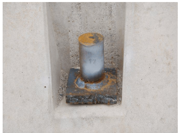
Barrier No. 4 Traffic Side Downstream
