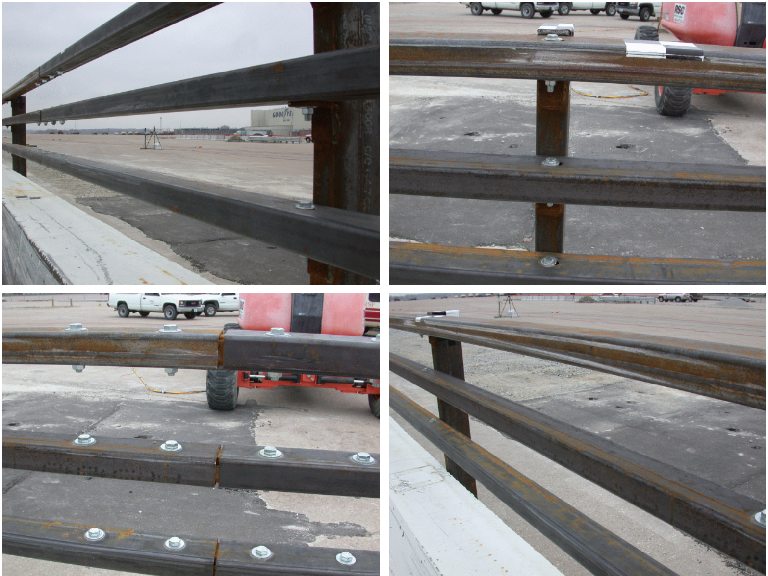
Figure 28. System Damage, Test MOBR-1
