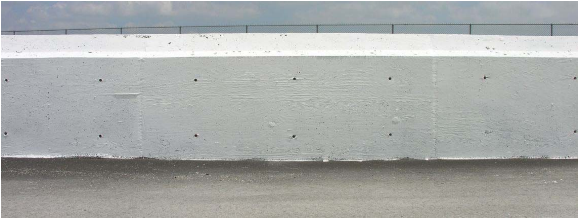
Figure 60. TL-5 Concrete Median Barrier
