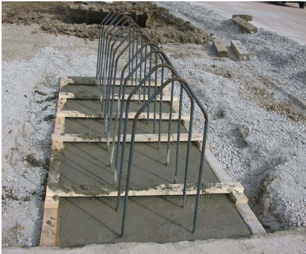
Figure 56. Reinforcement and Casting of Footer with Barrier End Section Stirrups
