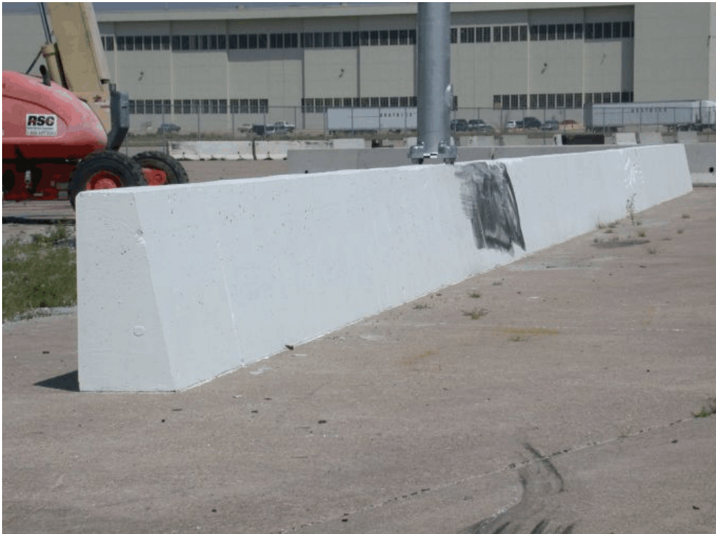
Figure 50. System Damage, Test No. ZOI-2
