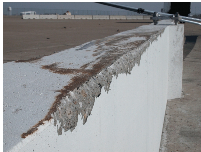
Figure 36. System Damage, Test No. ZOI-1
