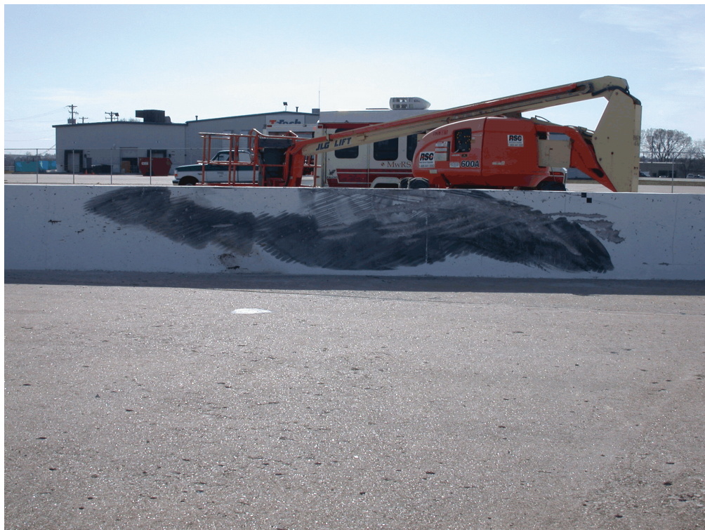
Figure 35. System Damage, Test No. ZOI-1
