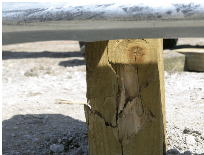
Figure 60. Post No. 6P Damage, Test SR-5
