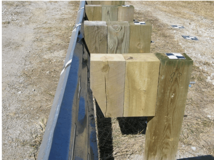
Figure 92. Post Nos. 6P through 8P Damage, Test SR-6
