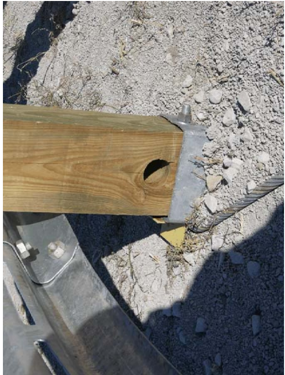
Figure 77. System Modifications, Test SR-6
