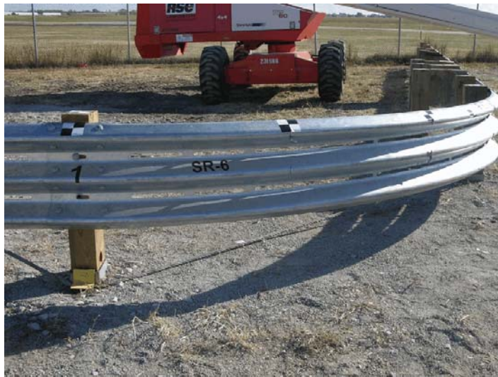
Figure 76. System Modifications, Test SR-2
