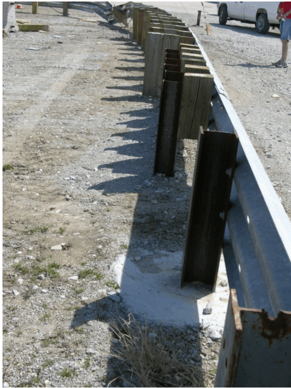
Figure 51. System Damage, Test SR-5
