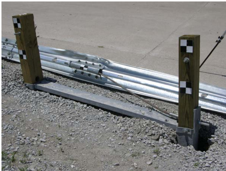
Figure 63. System Anchor Damage, Test No. LSC-2
