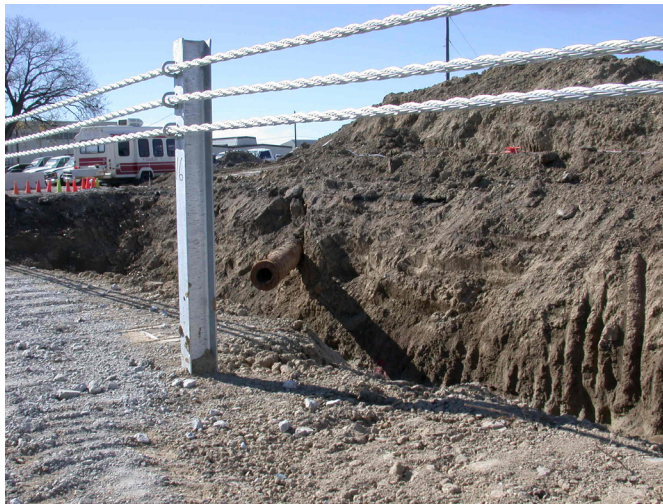
Figure 19. Three-Cable Guardrail System Adjacent to Slope
