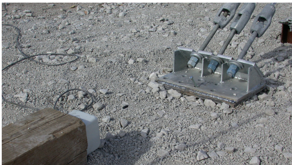
Figure 24. Three-Cable End Terminal Instrumentation
