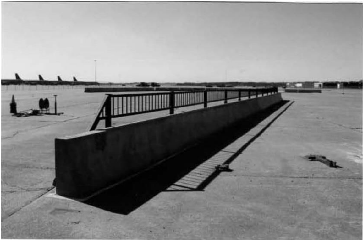
Figure 8. Minnesota Combination Traffic/Bicycle Rail [13]
