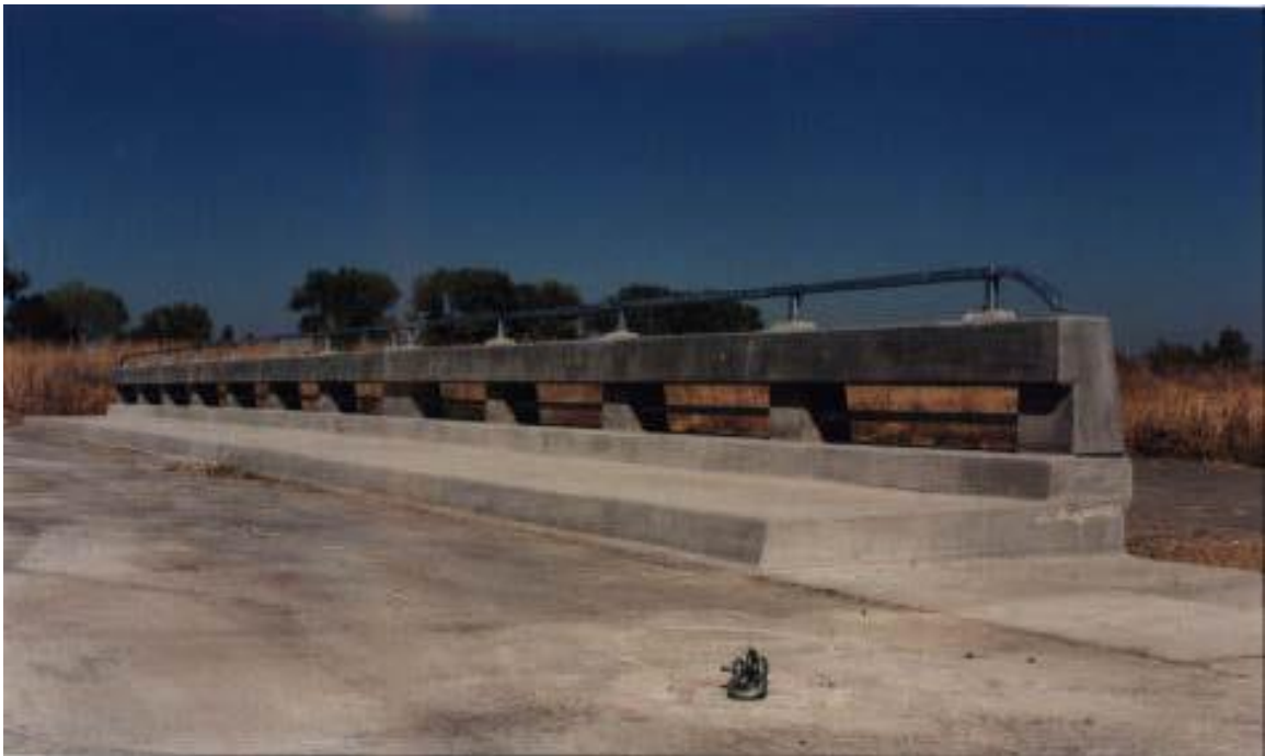
Figure 7. Type 80 SW Bridge Railing [12]
