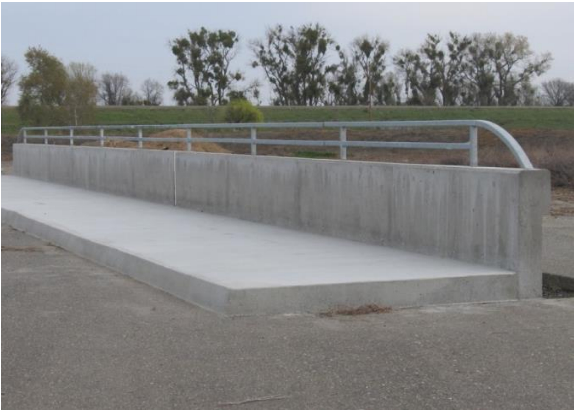
Figure 10. 732SW Bridge Rail [15]
