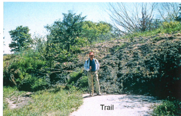
Fig. 61. Complex slide in Niobrara State Park (same site as Figure 59). Toe of the slide showing displaced materials and pieces of the underlying Niobrara Chalk carried downward by slide. Person for scale.
