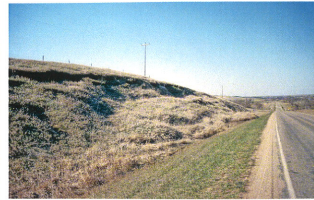
Fig. 28. Rock slump north of Bazile Mills along Nebraska Highway 13. Cretaceous System, Montana Group, Pierre Shale Formation. Typical landslide in Pierre Shale in a low sloping area. Slide materials have reached roadway several times previously.
