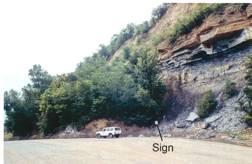
Fig. 4. Rock fall at Ponca State Park near the Missouri River boat ramp in Dixon County. Cretaceous System, Colorado Group, Greenhorn Limestone overlying Graneros Shale and Dakota Sandstone. Note small warning sign beside an unauthorized path.
