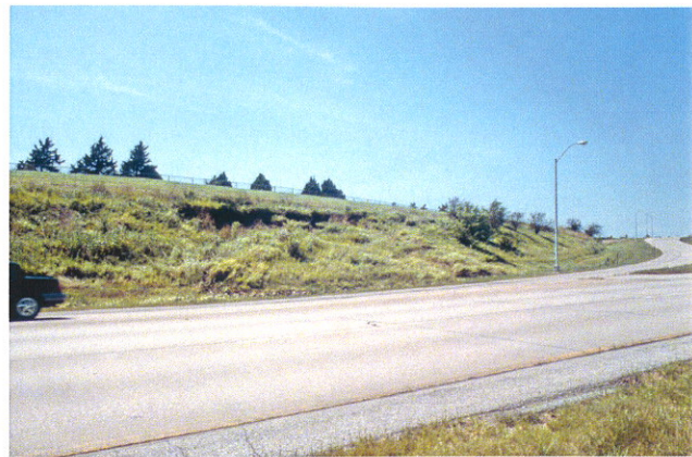
Fig 50. Earth slump in northwest Lincoln along Interstate I-180 in Lancaster County. Quaternary System, Pleistocene loess underlain by glacial deposits. Recurring slide.
