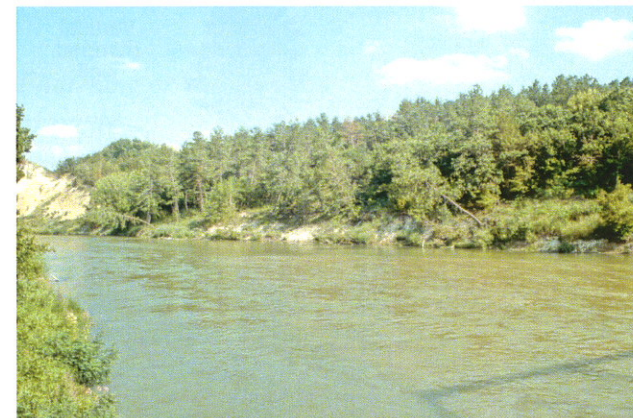
Fig. 63. Complex slide north of Johnstown (same site as Figure 62). Pierre Shale overlain by unconsolidated Pleistocene deposits. Tilted trees and materials from slide being eroded and carried downstream by the river. Professor John F. Shroder, Jr. and his students from University of Nebraska-Omaha's Geology Department have extensively studied site.
