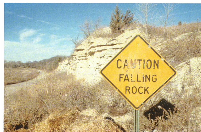
Fig. 6. Rock fall on county road near Gilead, Thayer County. Cretaceous Greenhorn Limestone overlying Graneros Shale.
