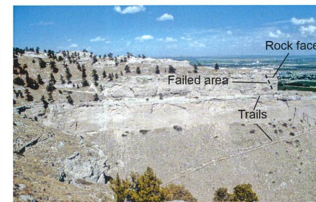
Fig. 12. Same site as Fig. 11 showing bluff and rock face before the rock fall. Hiking trails along the bluff are noted.
