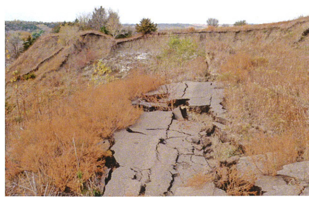
Fig. 25. Rock slump south of Niobrara. Same area as seen in Figs. 21-24 after 7 years. Old roadway is gradually moving downslope and breaking apart.
