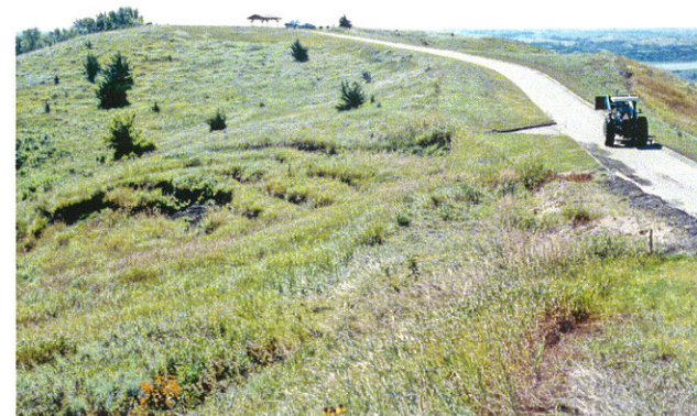
Fig. 36. Rock slump in Niobrara State Park, Knox County. Cretaceous System, Montana Group, Pierre Shale Formation. Slide scarp is approaching a park road. The entire park is underlain by Pierre Shale. Avoiding and mitigating slides in park is an ongoing project for park's maintenance department. Park is most affected by slides during periods of excessive precipitation in late winter and early spring.
