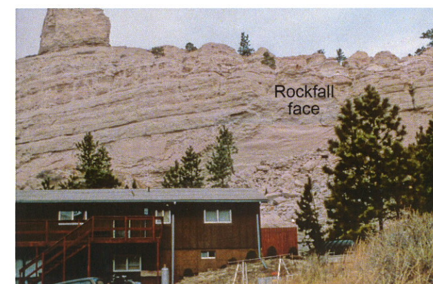
Fig. 9. Same site as Fig. 8 showing cliff behind the home and debris from the rock fall. Photo by John F. Shroder, Jr.
