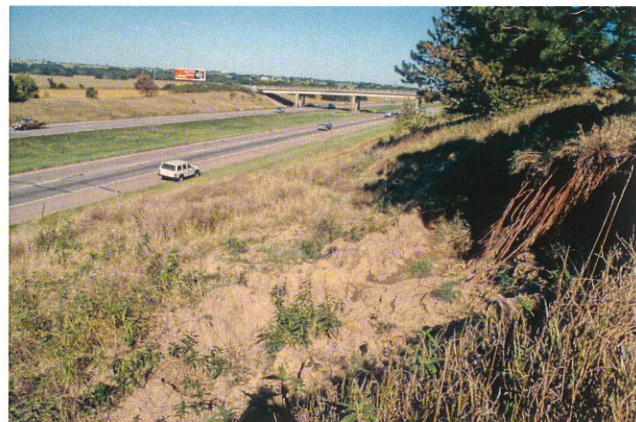
Fig. 42. Earth slump along Interstate 80 near Emerald, Lancaster County. Quaternary System, Holocene Series, Pleistocene loess with a possible paleosol underlain by Lower Cretaceous System, Dakota Group shale and sandstone deposits. Recurring slide, first noted a few years after I-80 was opened.
