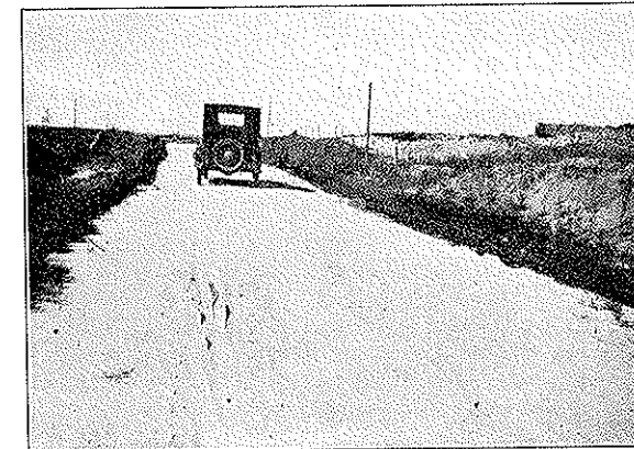
Figure 22. A Sandhill Road Southeast of Alliance, Surfaced With Magnesia Rock.
