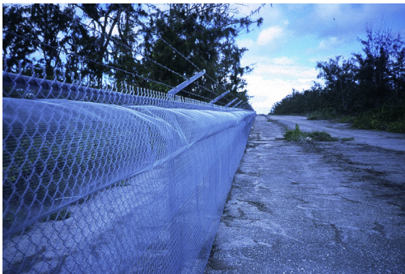
Fig. 5. Example of a permanent brown tree snake barrier attached to a chain link fence. Wire mesh prevents crossing through the fence and the wire mesh bulge creates an overhang the snakes cannot climb over. (Photo by R. Engeman).
