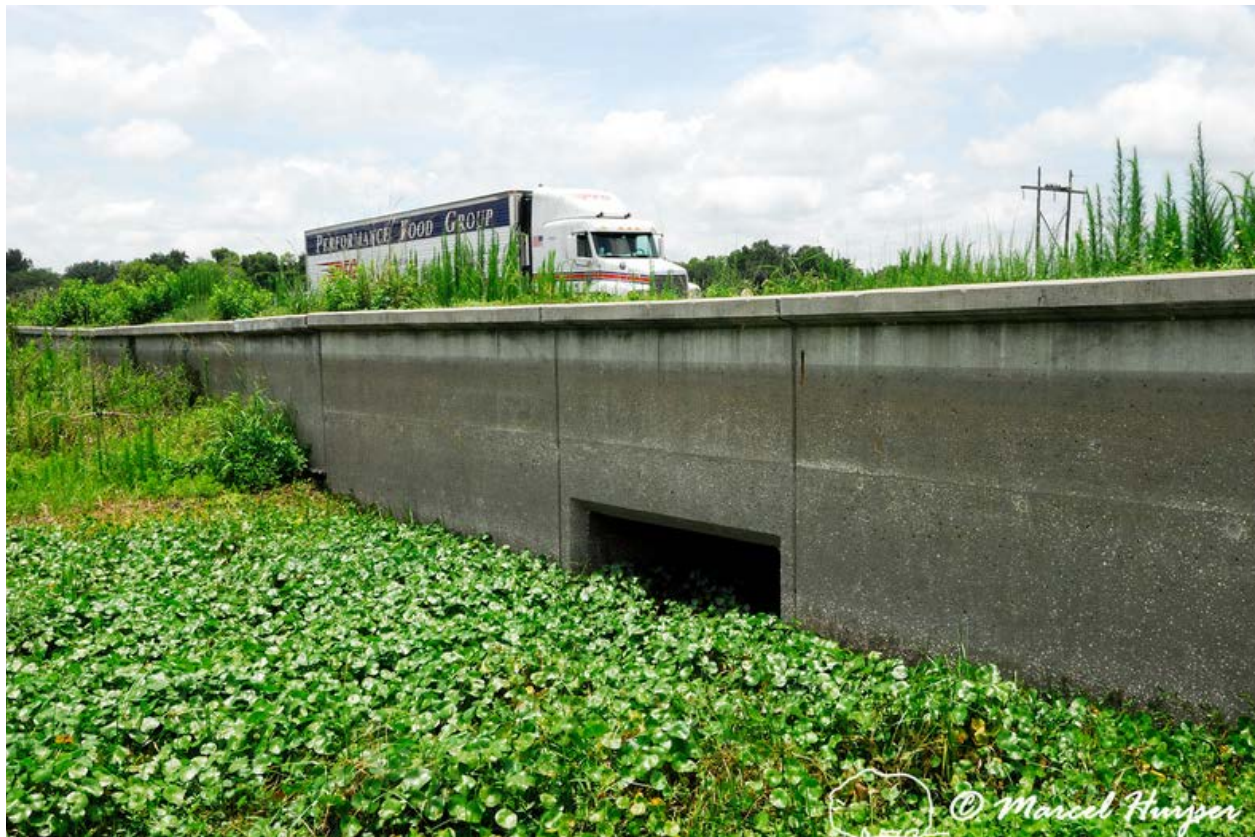
Figure 22: Underpass and barrier wall for reptiles, amphibians and small mammals, U.S. 441, Paynes Prairie Ecopassage, south of Gainesville, Florida, USA.
