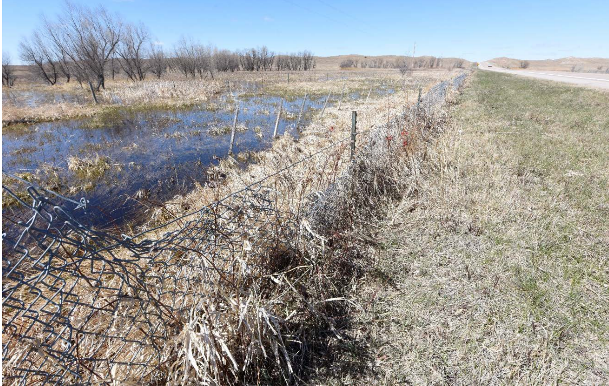
Figure 11: Fence detached from top wire and posts (Twin Lakes), April 2016.
