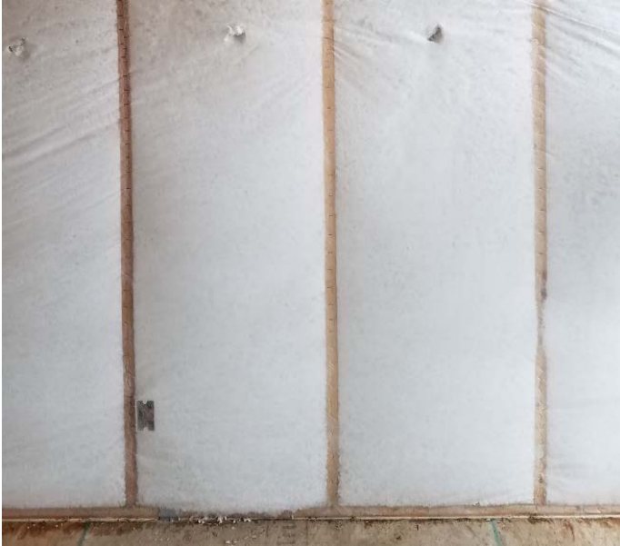
Figure 3.3 Exterior Wall Blown-in Insulation Verification
