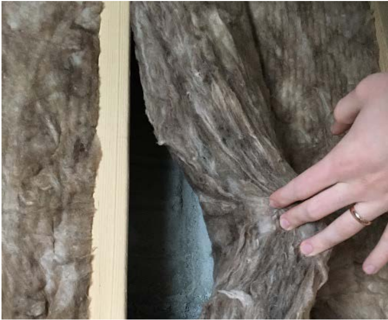
Figure 3.1 Basement Wall Fiberglass Batt Insulation Verification
