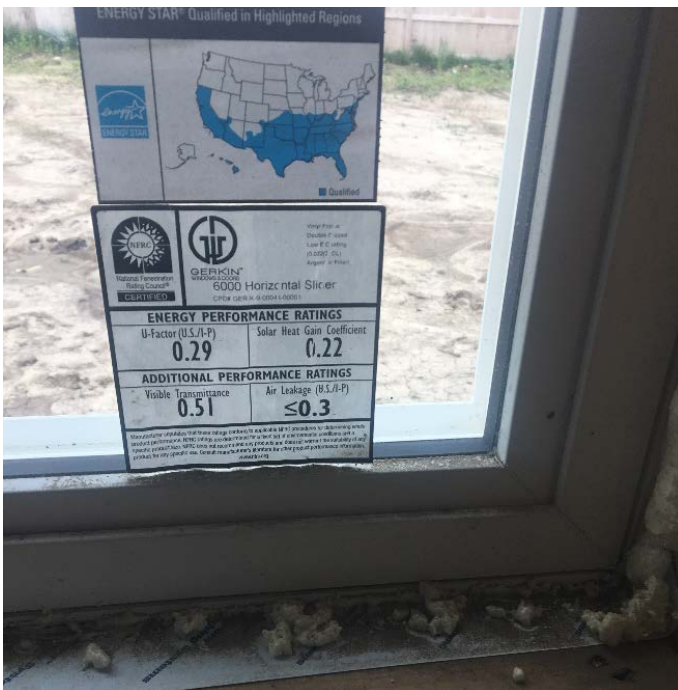
Figure 3.4 Window U-factor Verification
