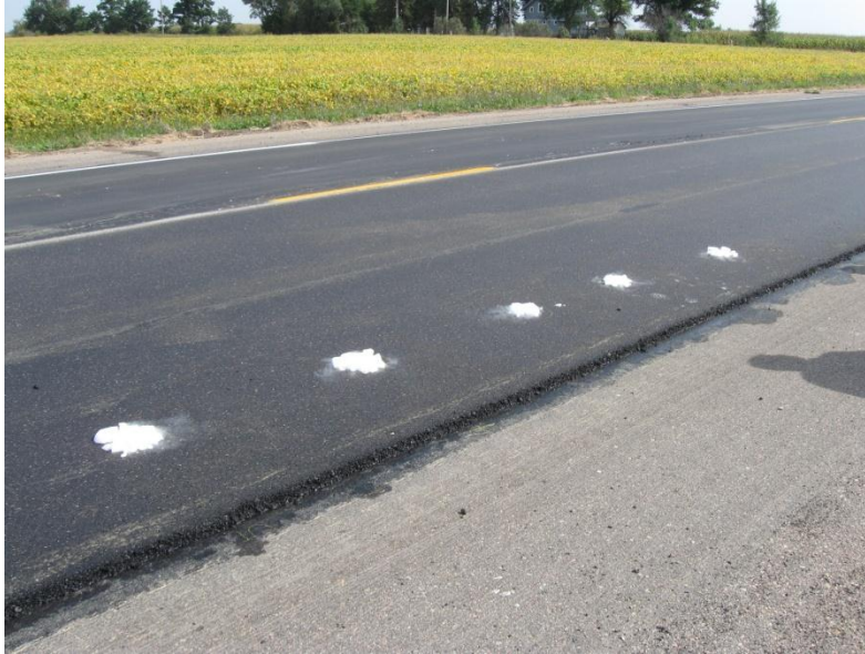
Figure 2.1. Dry ice cools the hot pavement
