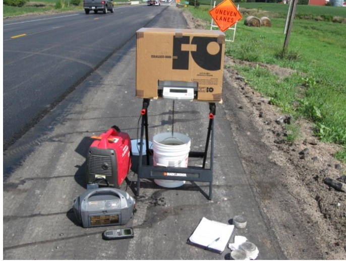
Figure 2.4. On-site set up for core measurements
