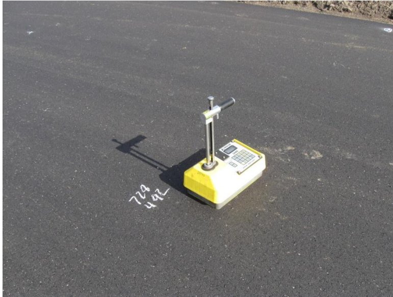
Figure 2.2. Nuclear Gauge is shown measuring density
