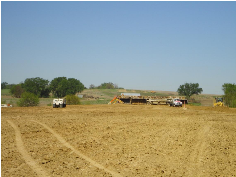
Figure 3.7. Platteview Intersection Site
