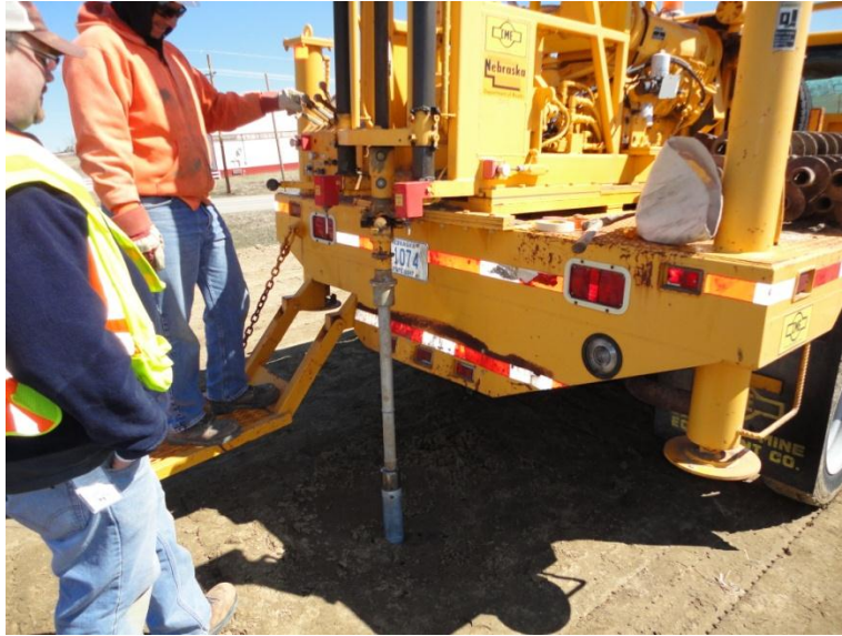
Figure 3.1. Shelby Tube driven in the ground
