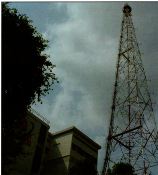
Cell phone towers work with your cell phone network so you can talk while on the road.
