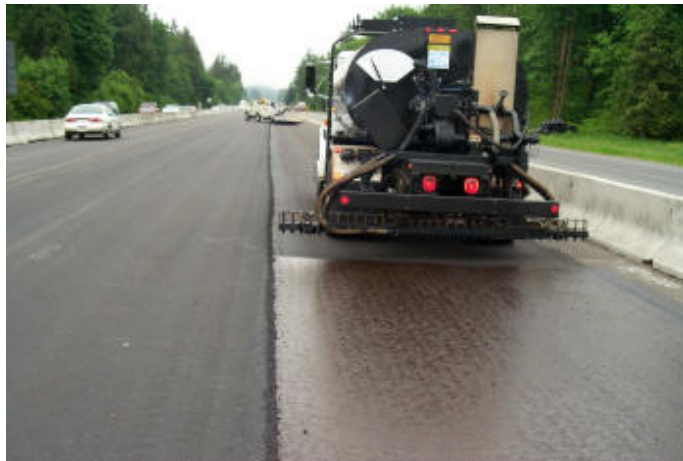
Figure 1-1. Typical tack coat applications.
