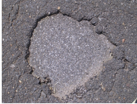
Figure 2-1. Delamination distress.
