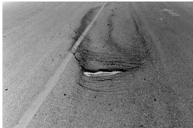
Figure 2-2. Slippage cracking.
