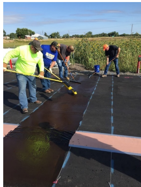
Figure 4-4. Distributing tack coat emulsion on the section.
