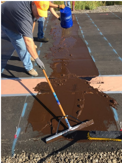
Figure 4-4. Distributing tack coat emulsion on the section.
