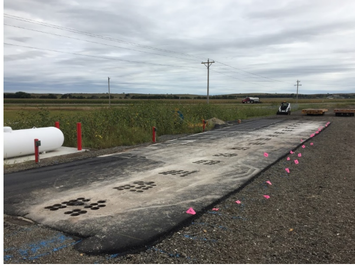
Figure 4-11. Coring 6-in. diameter samples.
