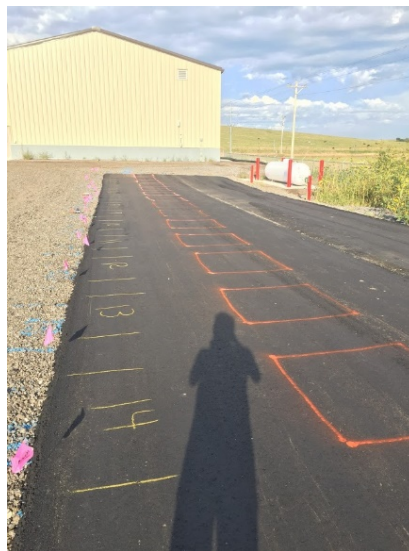
Figure 4-10. Marking coring areas out of wheel path.
