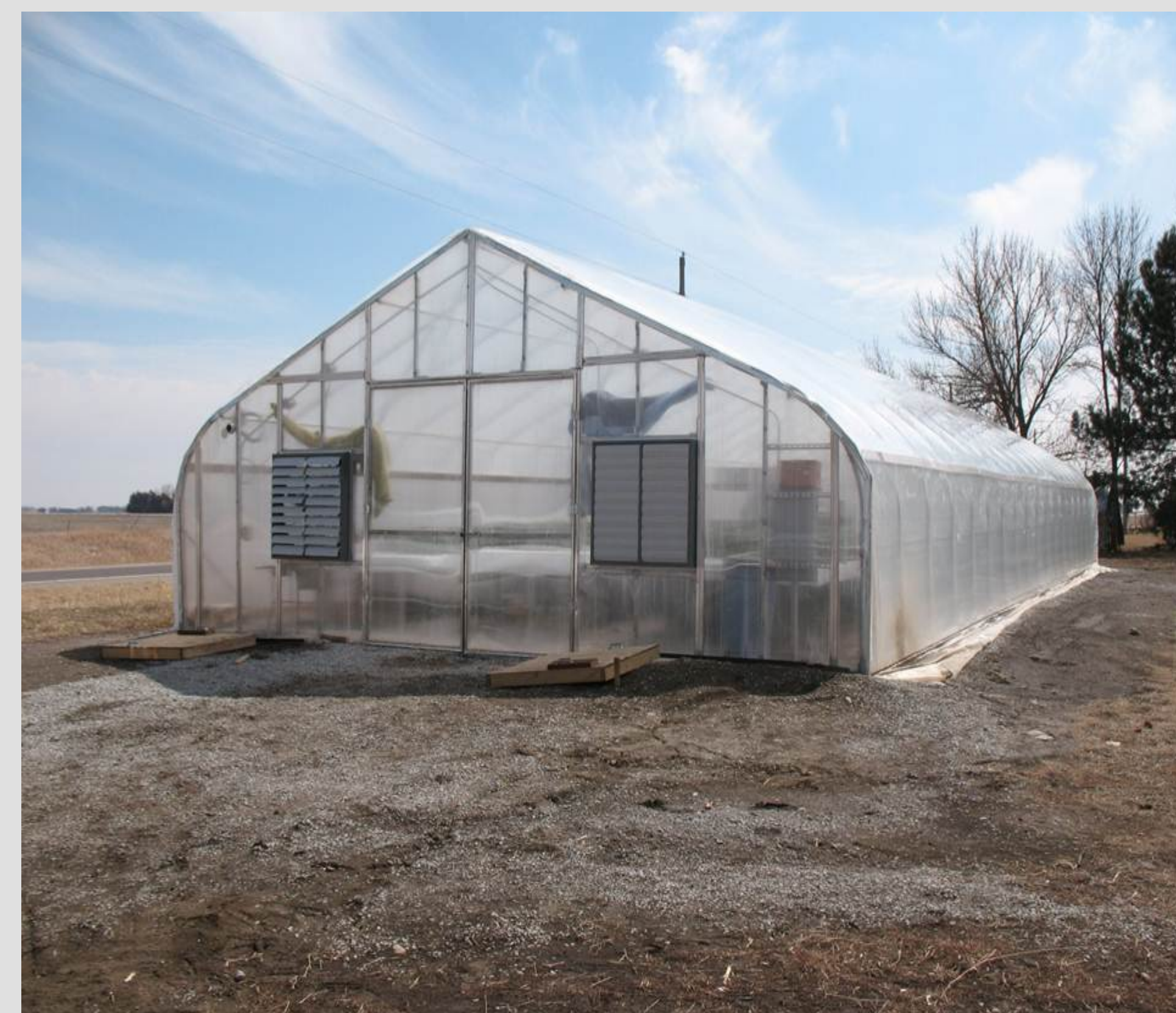
Figure 1. Double polyethylene heated high tunnel with acrylic end walls.
