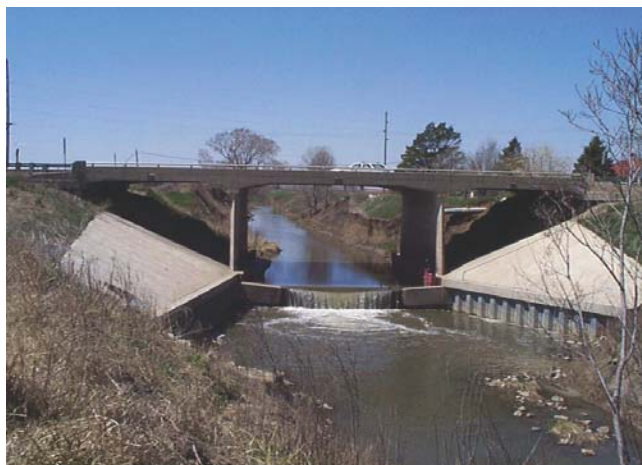
Figure 19. Drop structure at S Logan Cr at N15 (ER-12).
