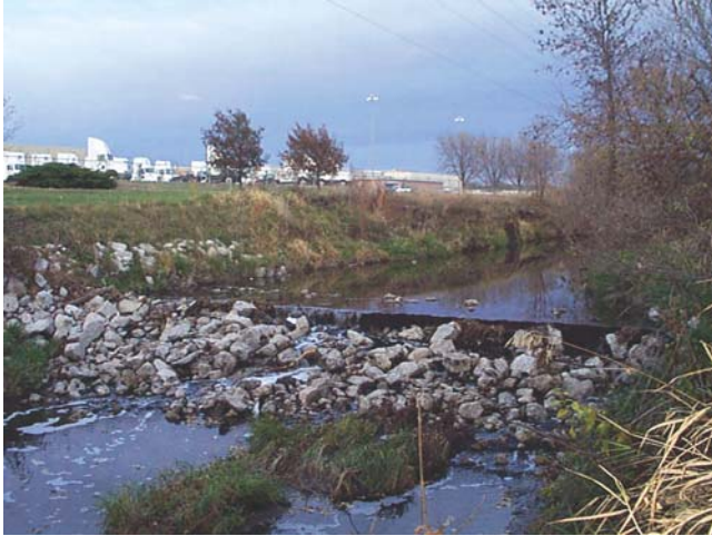
Figure 26. Grade-control structure on Beal Slough upstream from Link 55W (SC-H).
