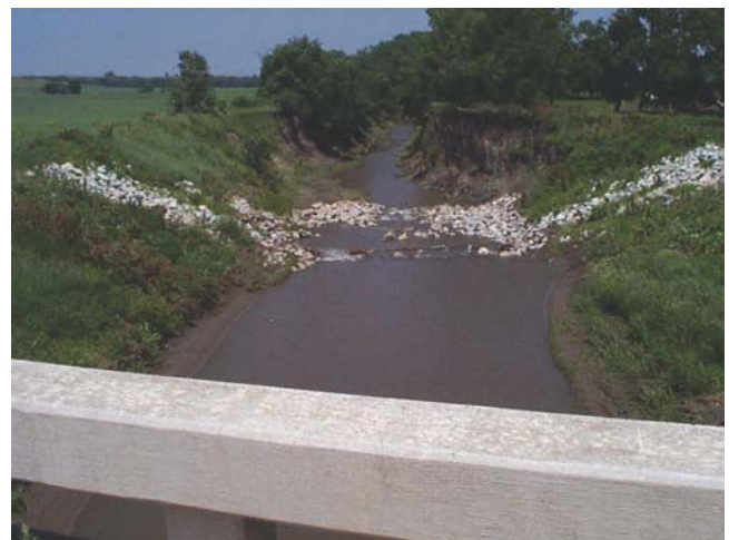
Figure 16. Looking downstream at grade-control structure on Skull Creek at PRT-5.
