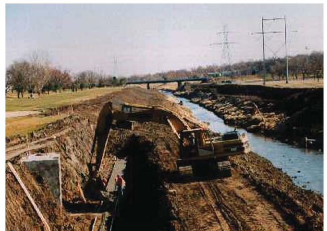
Figure 12. Channel and levee construction, Big Papillion Creek (photograph from the Papio-Missouri River Natural Resources District).
