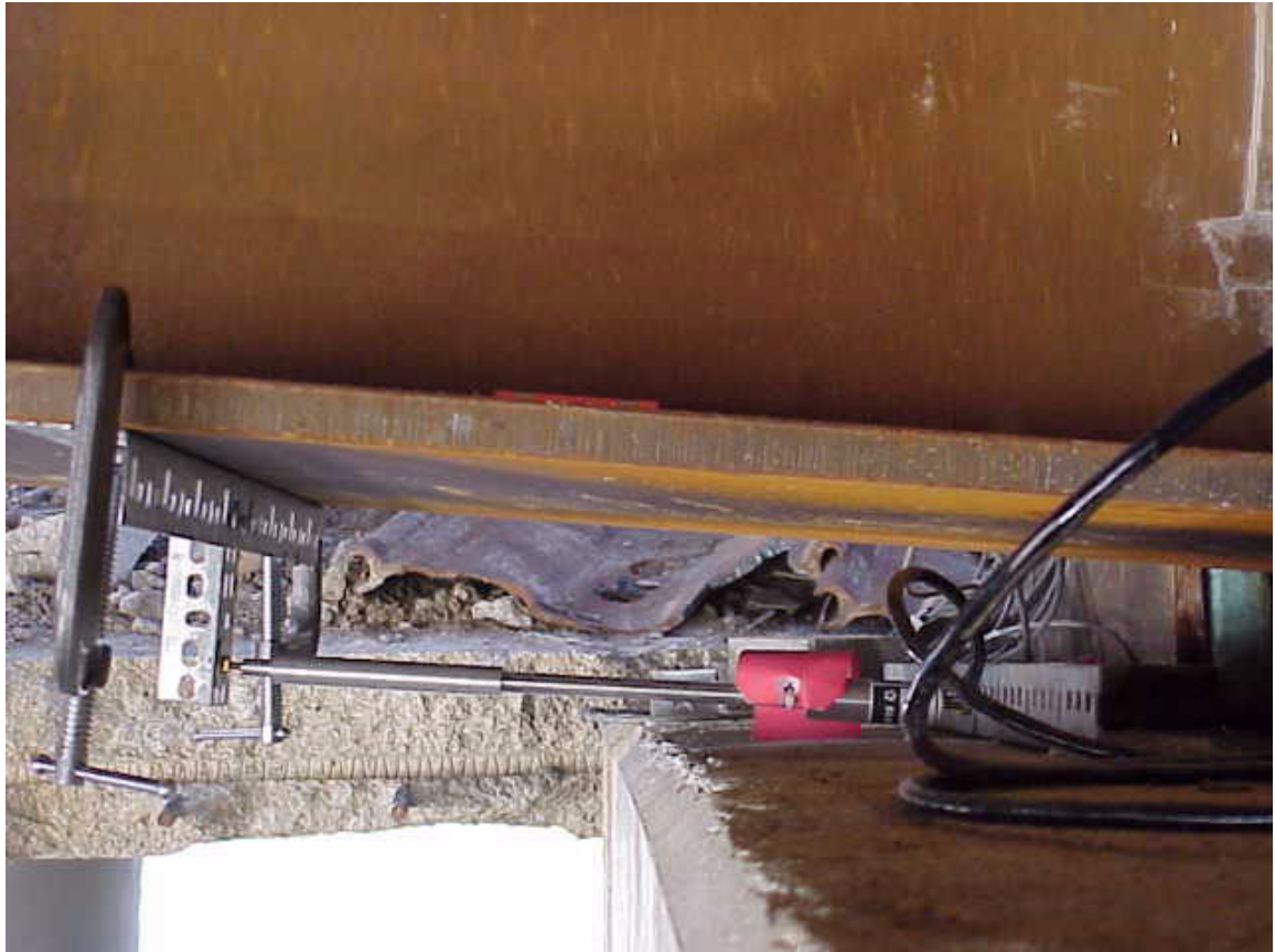
Figure 3-37: Crackmeter connected to girder flange
