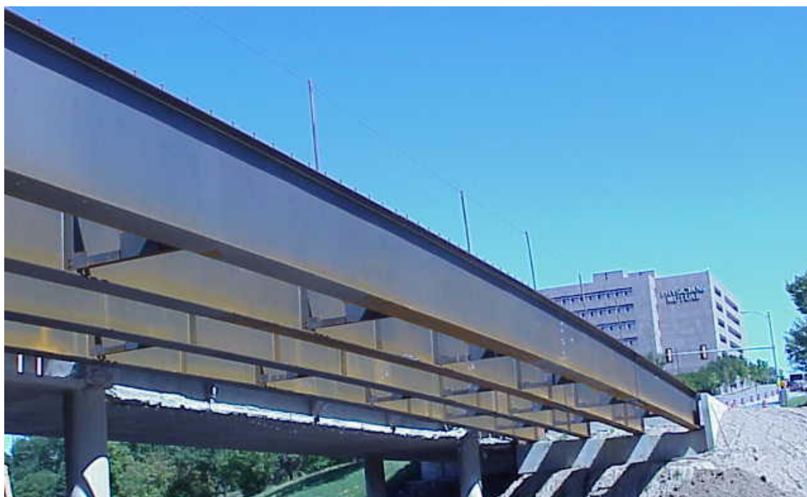
Figure 3-12: All four girders for East span in place.
