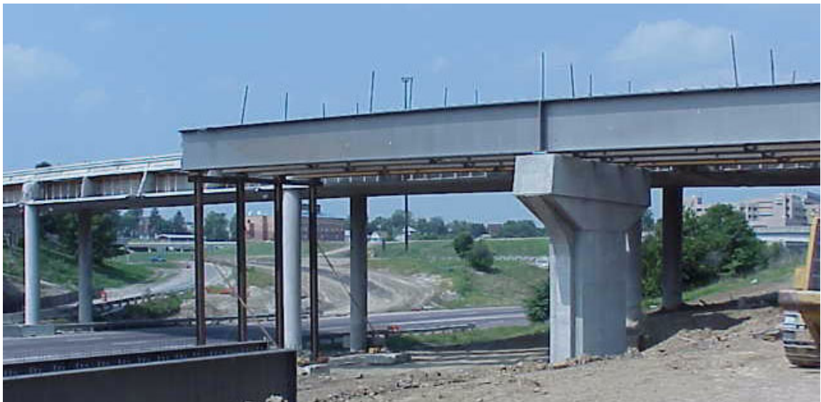
Figure 3-10: Girder sections E3, G3, H3, and J3 placed over the pier
