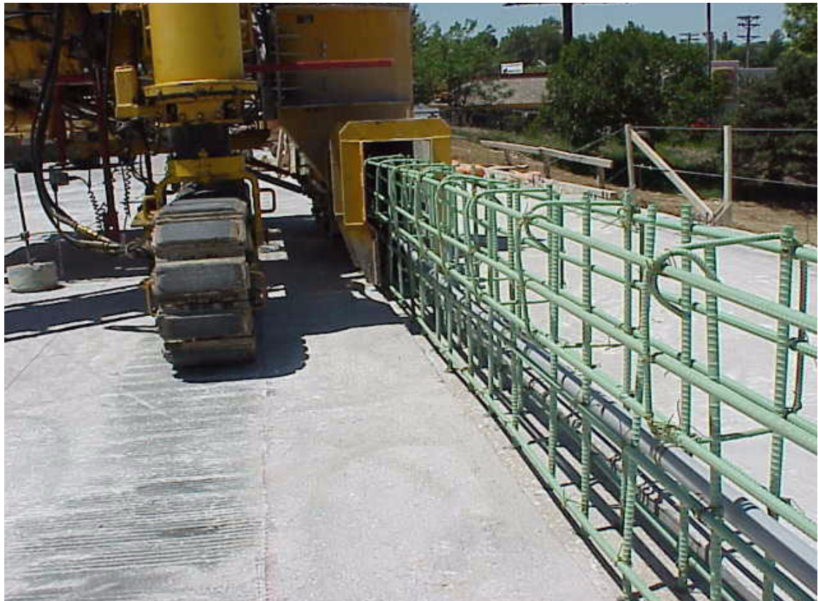
Figure 3-28: Phase II permanent barrier before casting. Note dowels epoxied into deck
