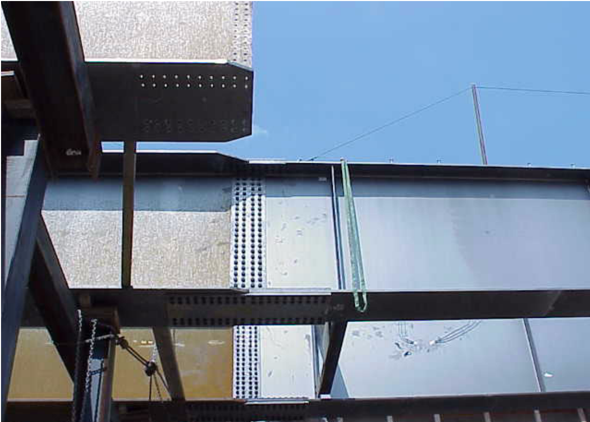
Figure 3-14: Girder splice
