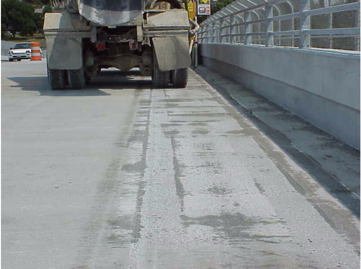
Figure 3-31: Finished permanent barrier. Note truck on bridge is grinding surface.
