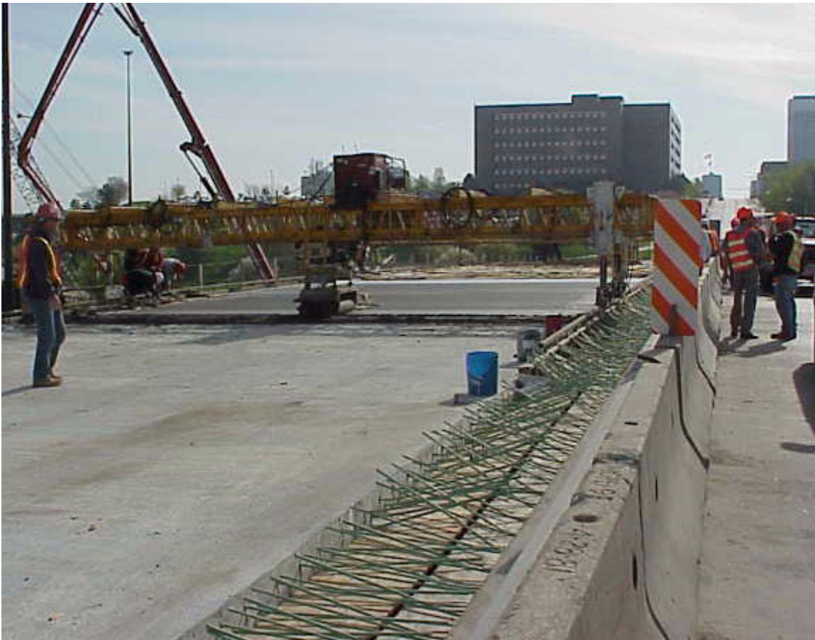
Figure 8-3: Transverse Reinforcement Bent to Allow Clearance
