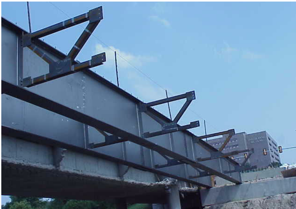
Figure 3-11: Girder sections 4 and 5 of the East span
