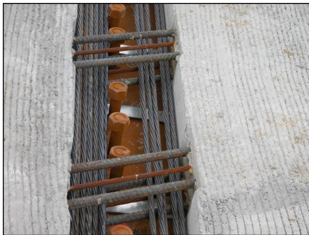
Figure 1.2: Threading post-tensioning strands (left) and conflicts between deck reinforcement and shear connectors (right)
