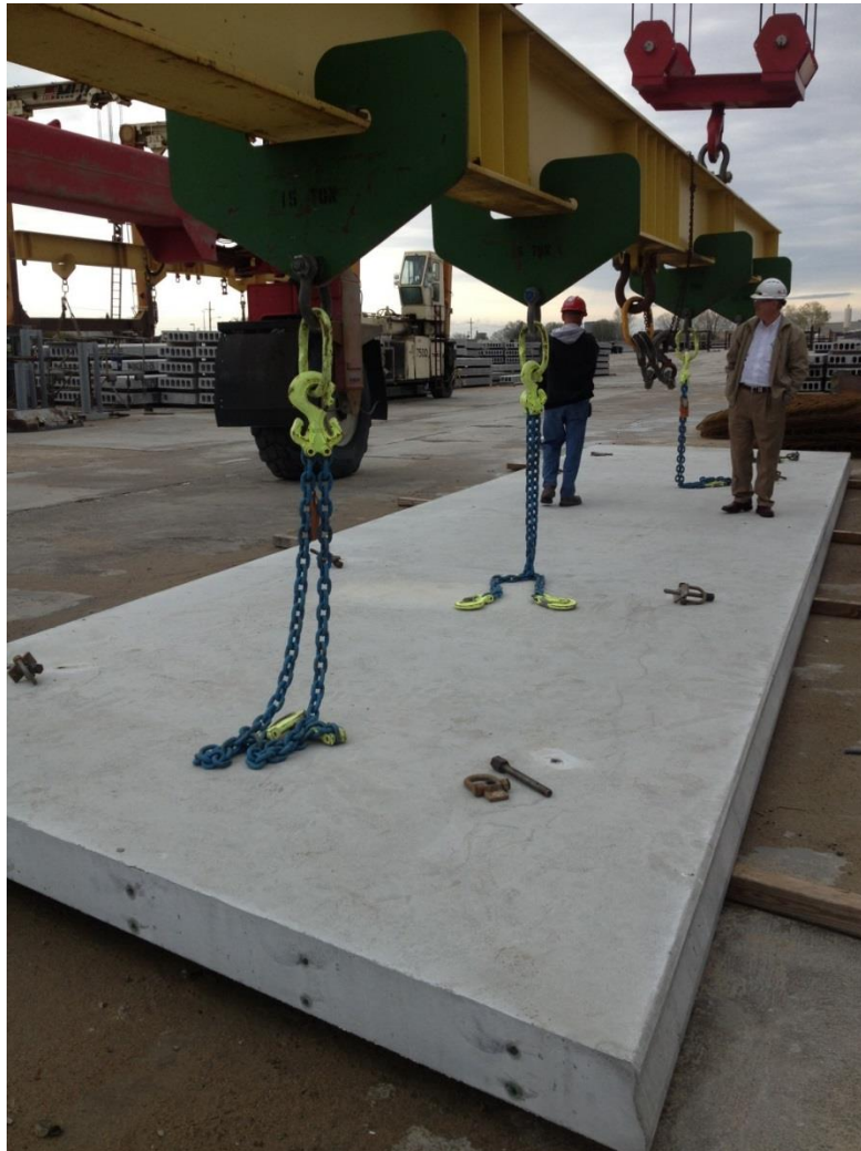
Figure 6.6: Demonstration panel before lifting and the spreader beam
