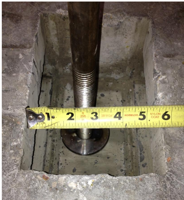
Figure 5.28: The two pockets prior to grouting
