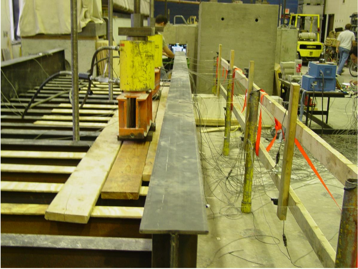
Figure 4-35. Instrumentation Installed on Top Flange of Plate Girder
