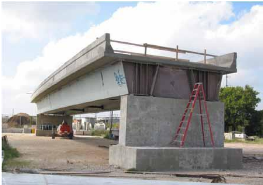
Figure 1-1. FSEL Twin Box-Girder Bridge [Source: FHWA Report No.: FHWA/TX-10/9-5498-1]
