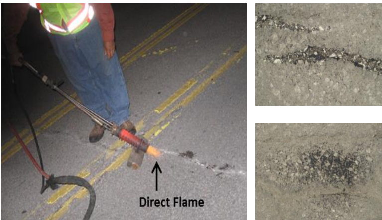
Figure 1.1 Direct flame problem in hot air blasting (heat lance) causing soot residues
