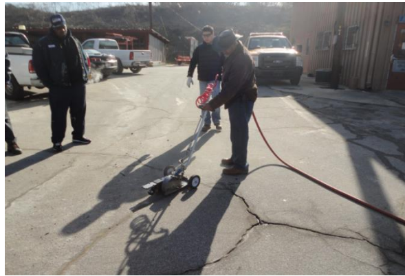
(c) Testing by GDOT crew
