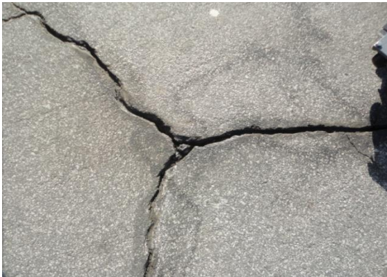
(b) Routed cracks
