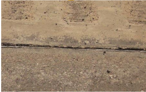
(a) CCD : Cleaned crack
