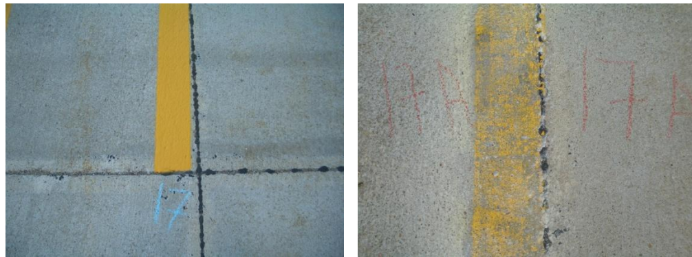
Figure 6.8. Concrete pavement condition before (left) and after (right) 12 mils oil-based paint has been removed by dry ice blasting
