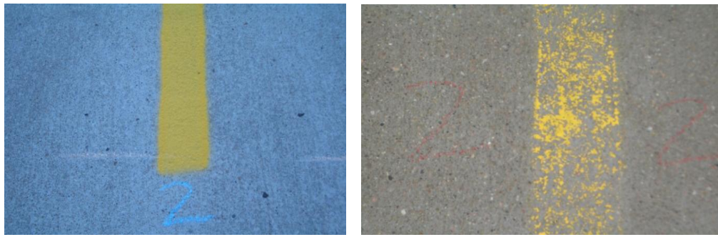
Figure 6.7. Concrete pavement condition before (left) and after (right) 10 mils water-based paint has been removed by dry ice blasting
