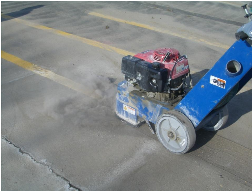
Figure 2.3. Grinder removing paint on asphalt pavement
