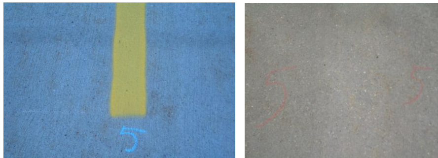
Figure 6.18. Concrete pavement condition before (left) and after (right) paint has been removed by chemicals
