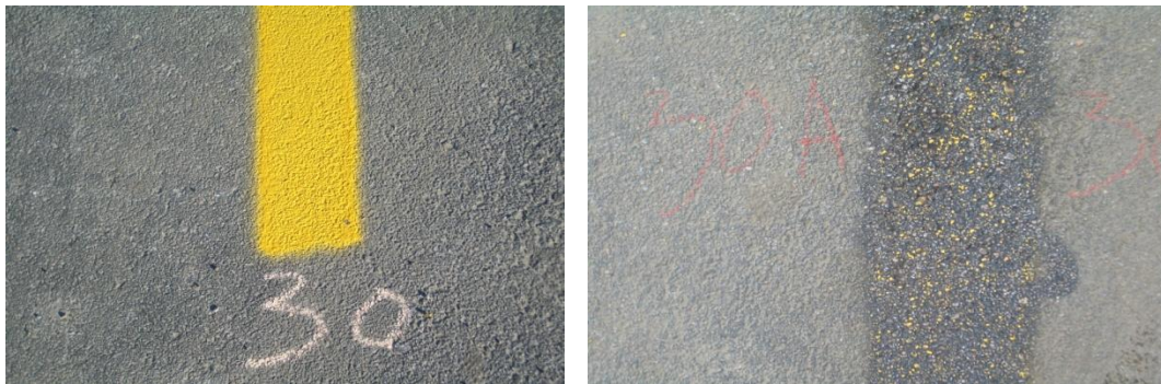
Figure 6.9. Asphalt pavement condition before (left) and after (right) paint has been removed by dry ice blasting
