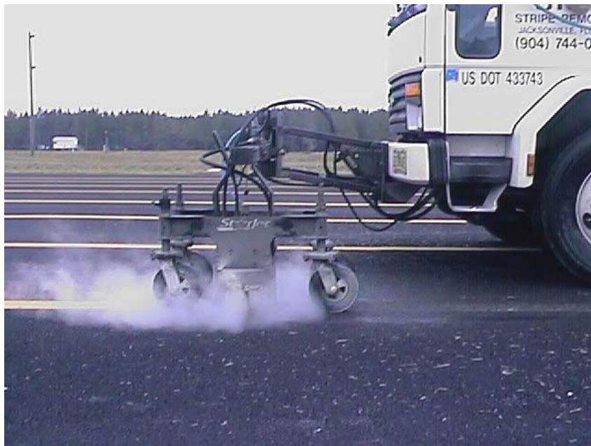
Figure 2.2. High pressure water jet water blasting pavement marking
