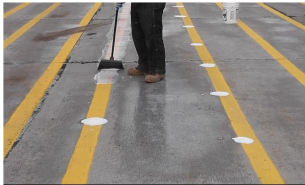
Figure 6.16. Applying the chemicals on the markings
