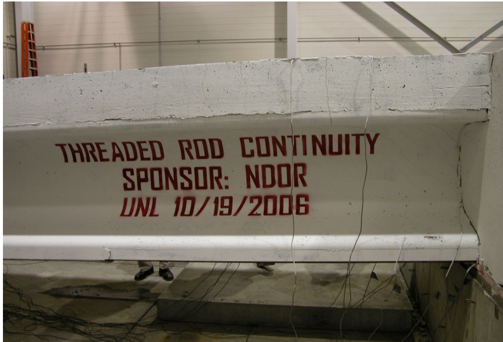
Figure 3.3.20: Final Flexural-shear Crack near the Pier, P = 324 kips
