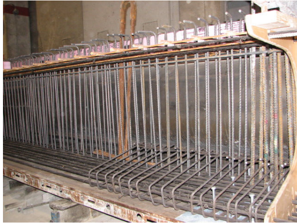
Figure 2.5.1: Shear and confinement reinforcement
