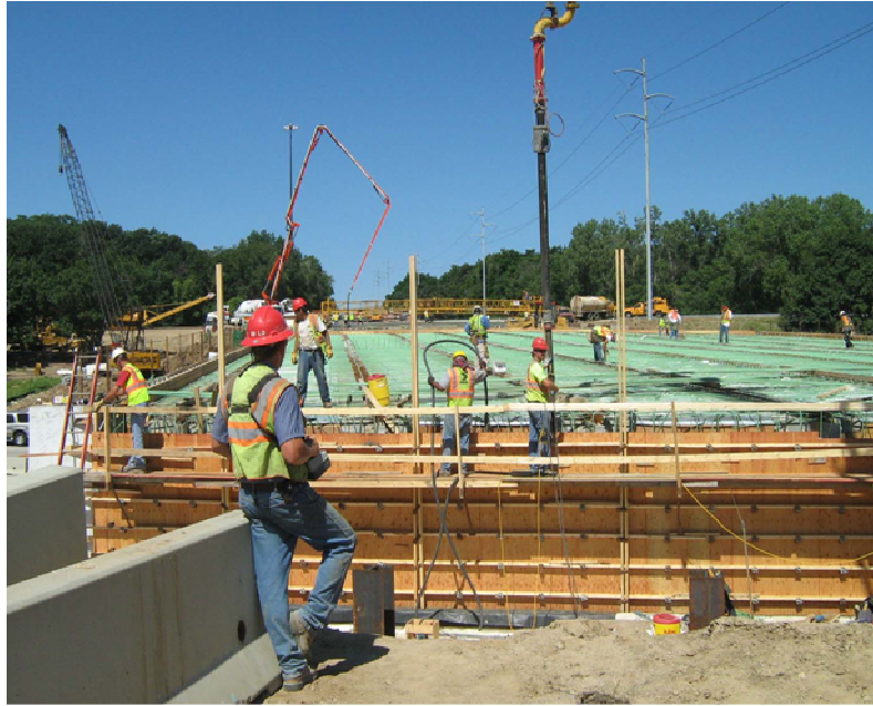
Figure A.12: Pouring of Concrete
