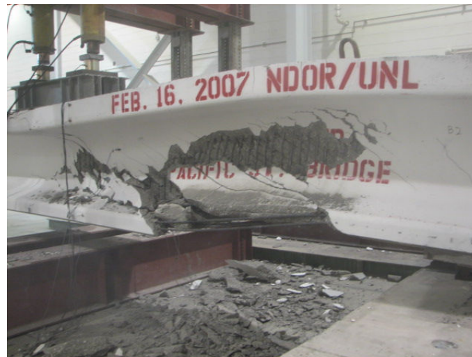
Figure 2.11.4.5: Immediately after shear failure
