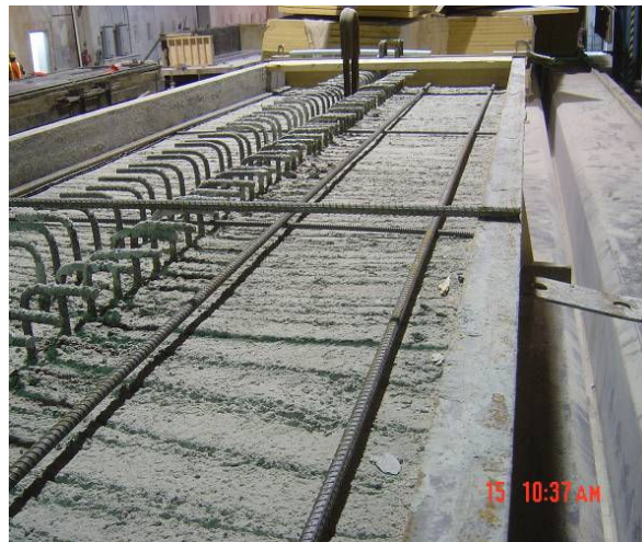
Figure 2.8.1: Longitudinal #5 deck reinforcement
