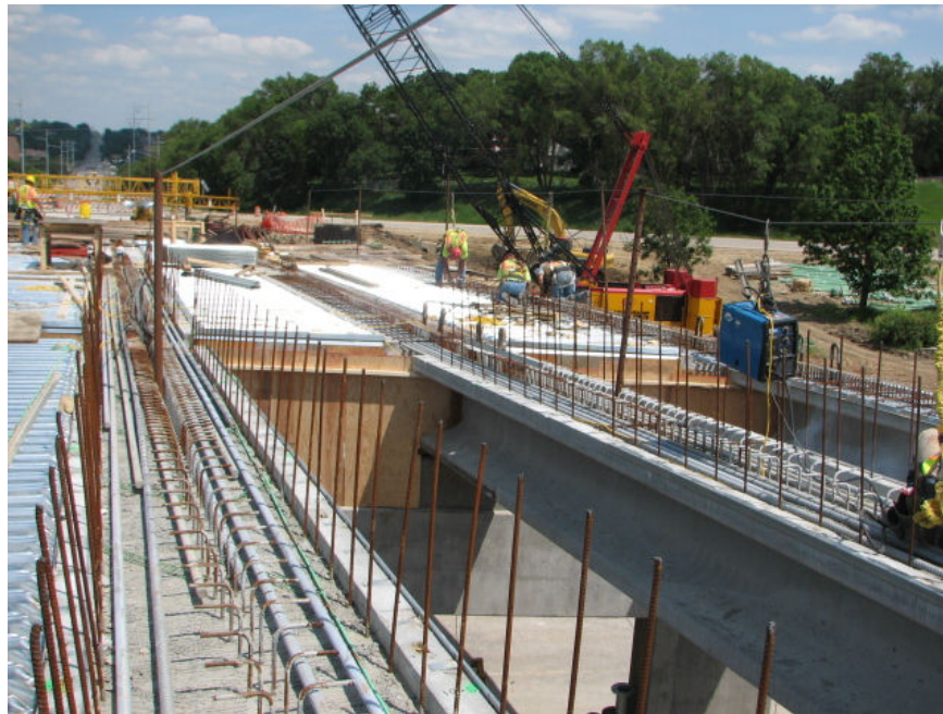
Figure A.3: Placement of Deck
