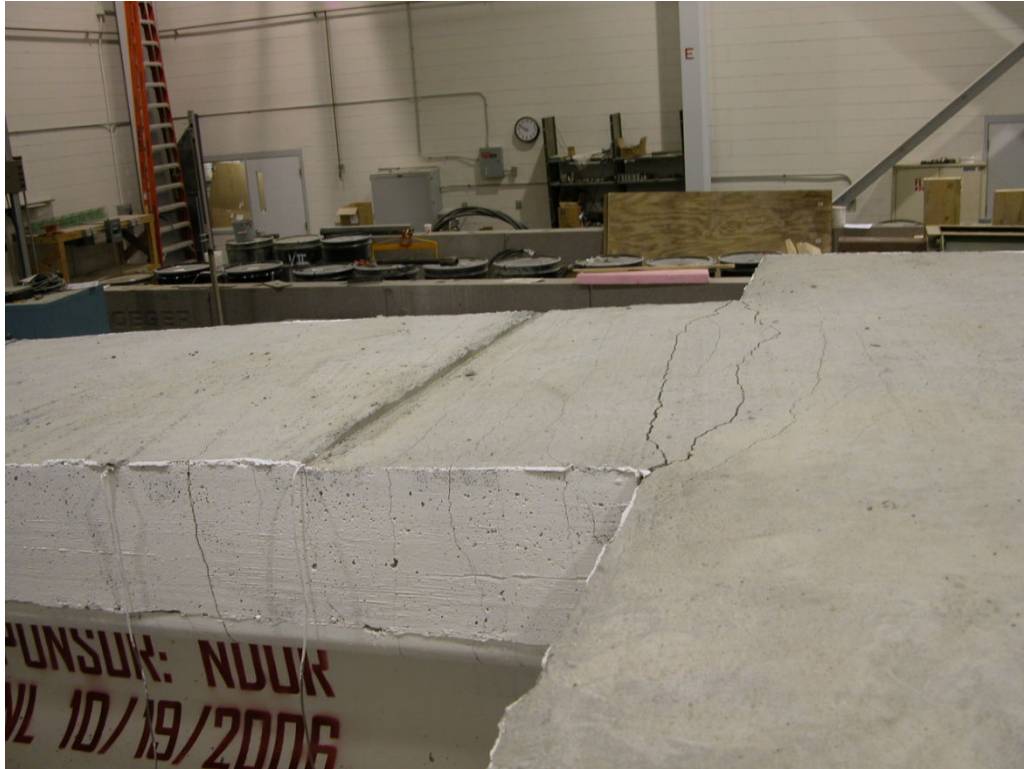
Figure 3.3.29: Crack on the Top at Failure
