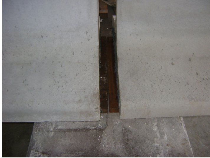
Figure 4.4.3: Placed girders with 4 inch gap
