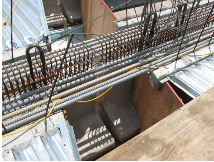
Figure A.4: Girders at diaphragm section
