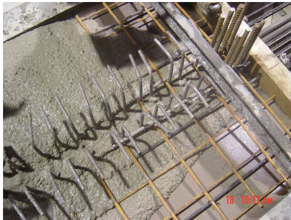
Figure 2.5.5: Pouring the girder using SCC
