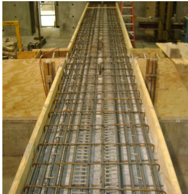
Figure 4.5.2: Placement of deck reinforcement
