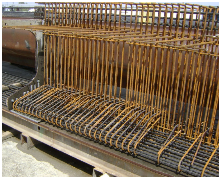
Figure 4.3.7: Placement of web and top flange reinforcement
