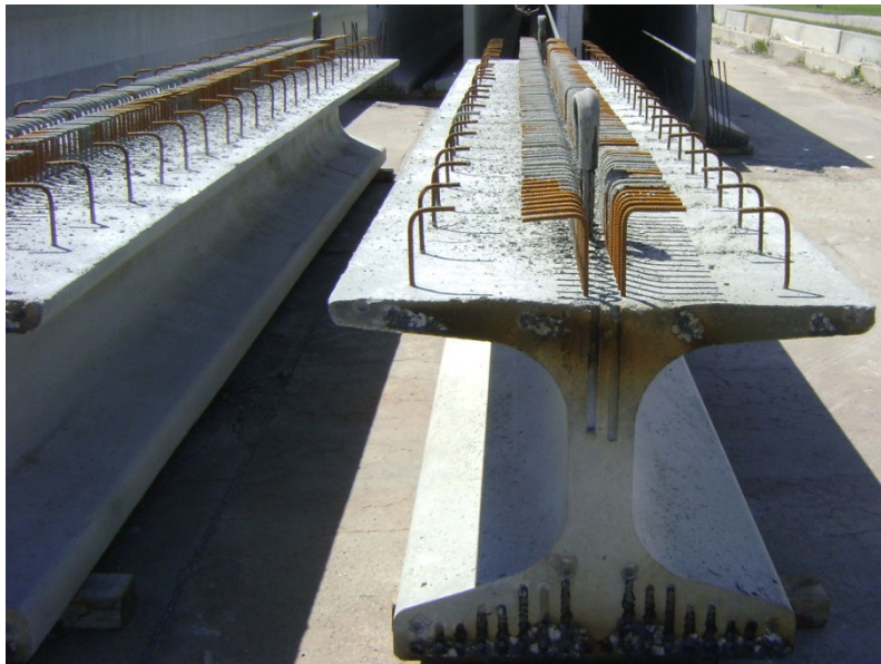
Figure 4.3.9: Girders after release
