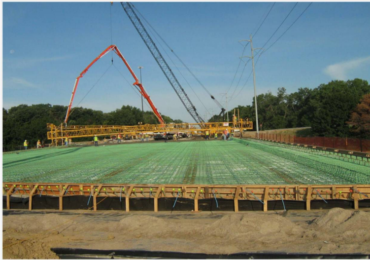
Figure A.5: Bridge construction
