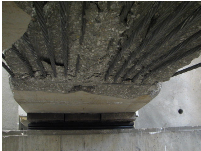
Figure 2.11.4.11: Confined flange non-failed
