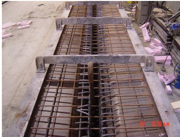
Figure 2.5.4: Top reinforcement
