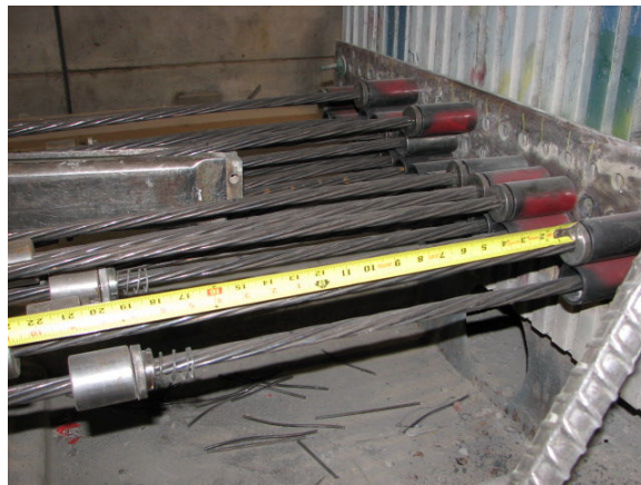
Figure 2.4.1.3: Mono-strand jacking
