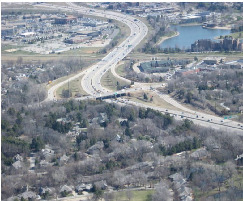
Figure A.1: Aerial View of Previous Bridge
