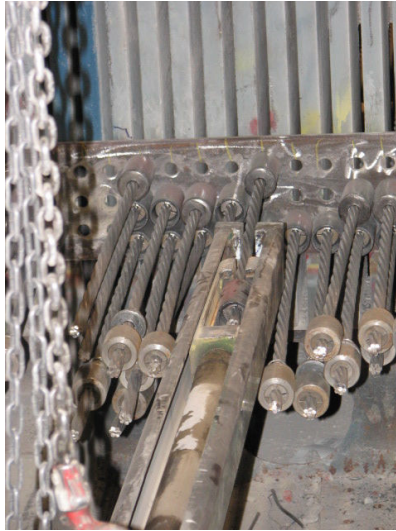
Figure 2.4.1.3: Mono-strand jacking
