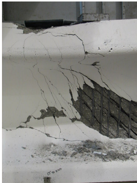
Figure 2.11.4.7: Flexure cracking at load point
