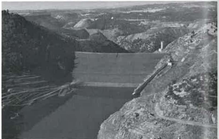
The Bureau of Reclamation suspended operation of New Melones Dam, a hydroelectric plant near Modesto, California, in the early 1990s due to six years of drought and a lack of significant precipitation. The low level of the reservoir was apparent in the fall of 1991, when this aerial view of the dam's upstream face was photographed. The intake structure is visible on the right side of the photograph. (Courtesy of the Bureau of Reclamation)
