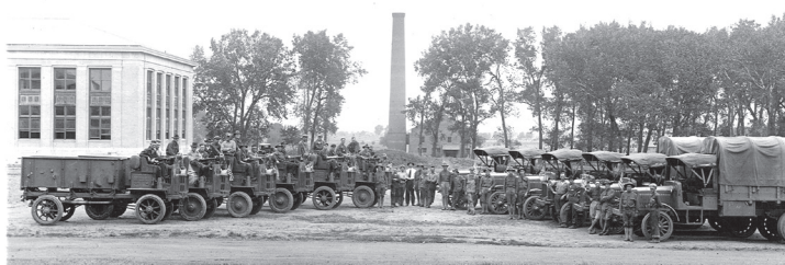
The building quartered WWI troops, a truck operator school, and caisson construction.
