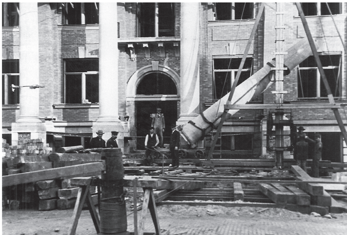
Pillars were brought to site on temporary rail tracks, as pictured here.
