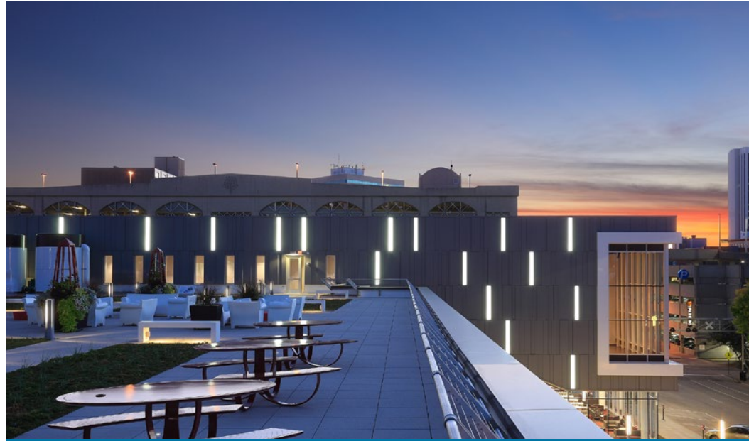
An outdoor area at the Downtown Library in Cedar Rapids, Iowa, is as functional as it is beautiful. The area, which is adjacent to the library’s green roof, has become popular for community events and weddings. Photo courtesy of Main Street Studio: Wayne Johnson.
