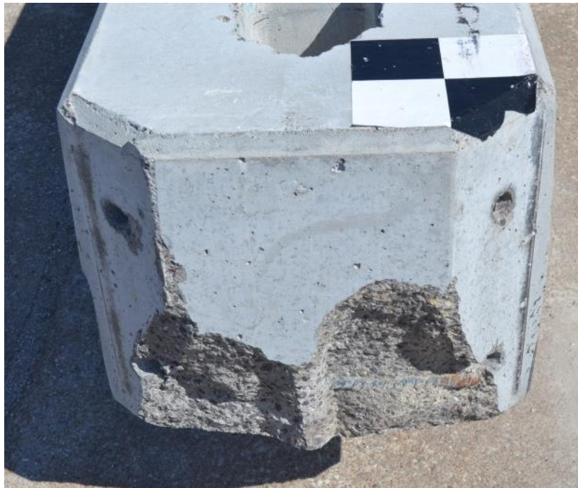
Figure 43. RESTORE Barrier Damage, After ACJ Removal, Test No. SFH-3 [20-21]
