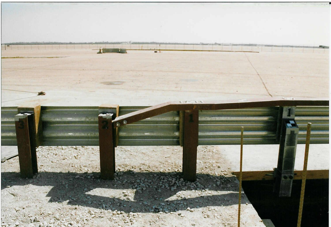
Figure 24. TL-4 Transition on Transverse Glue-Laminated Timber Deck [51-52]
