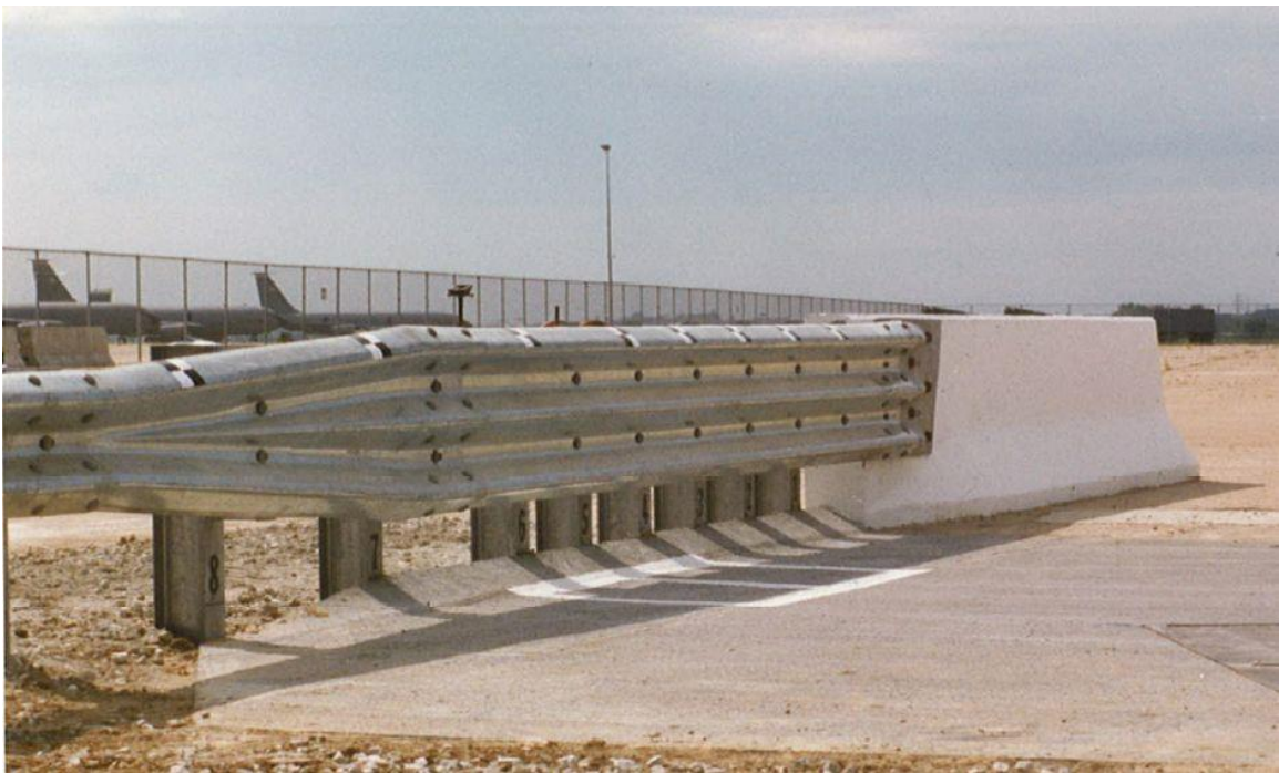
Figure 25. Horizontal Flare Rate of 6H:1V Barrier Toe [53-54]
