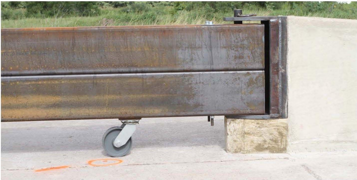
Figure 13. Final Design of the Emergency Opening System [34-35]
