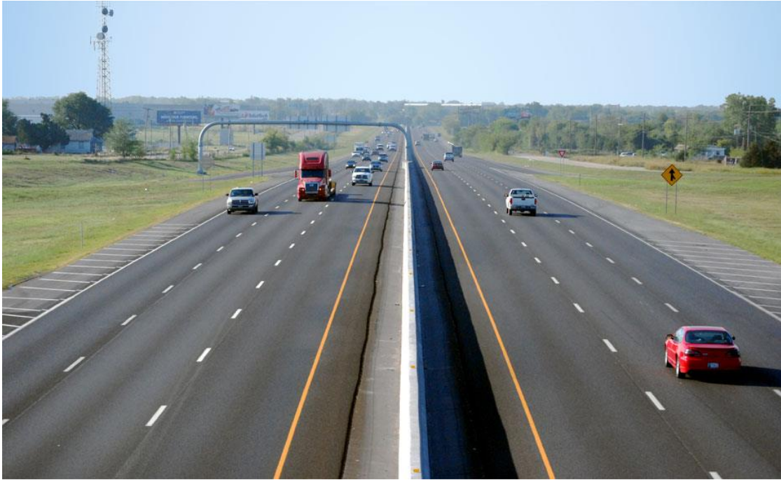
Figure 1. Double-Sided Concrete Barrier in Narrow Median [1]
