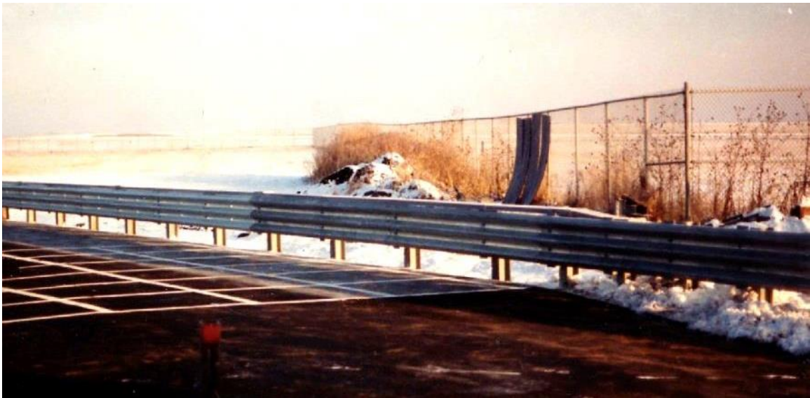
Figure 23. TBC-8000 Bridge Rail Transition [47-49]
