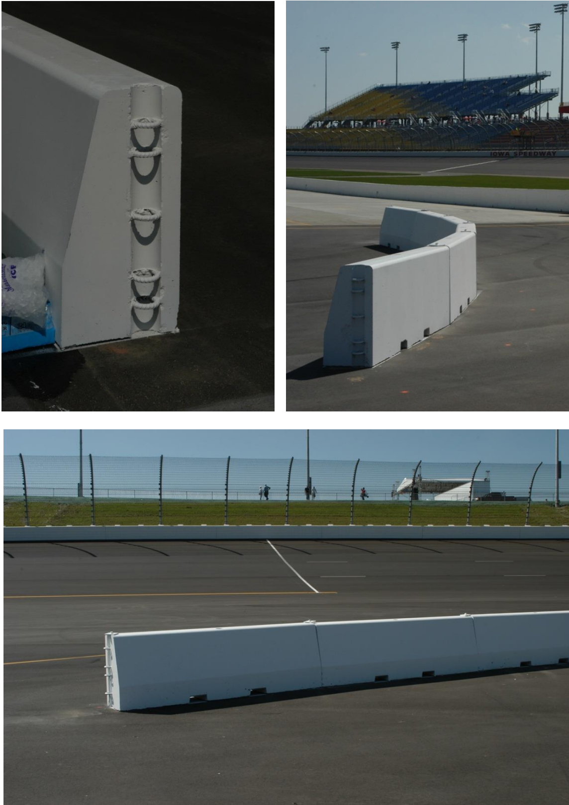
Figure 15. Portable Concrete Barrier Design for Iowa Speedway [39-40]
