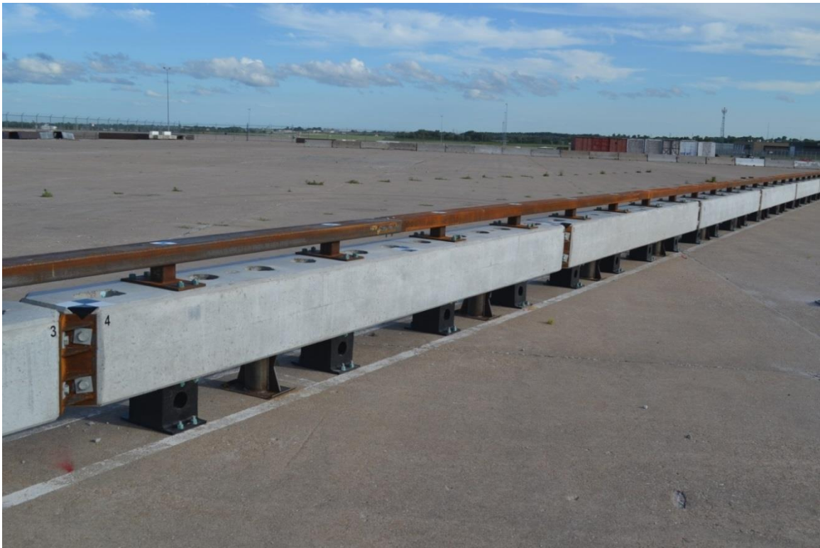
Figure 5. Overview of RESTORE Barrier
