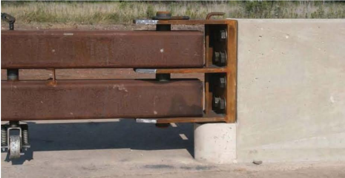
Figure 11. Original Emergency Opening System [33]
