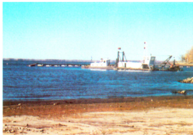
Fig. 9. Dredge clearing harbor and marina of sediment
