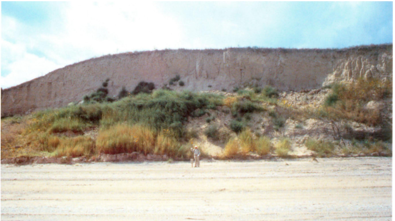
Fig. 30. Complex slide at site 12. Man is about 5.5 feet tall.
