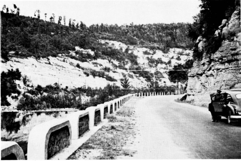
Figure 16. Road through a deep cut.
