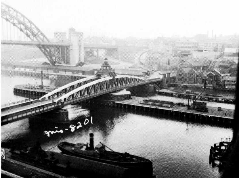
c. The housing is over the center of the swing span, which can be pivoted until it is directly over the wharflike structure.
