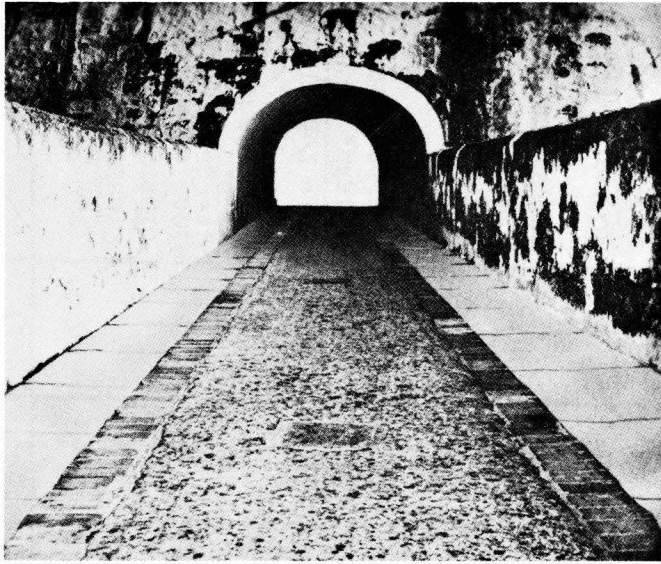
Figure 54. Concrete lined tunnel.
