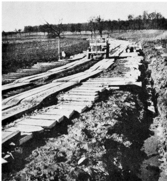
b. Plank road with a drainage ditch.
