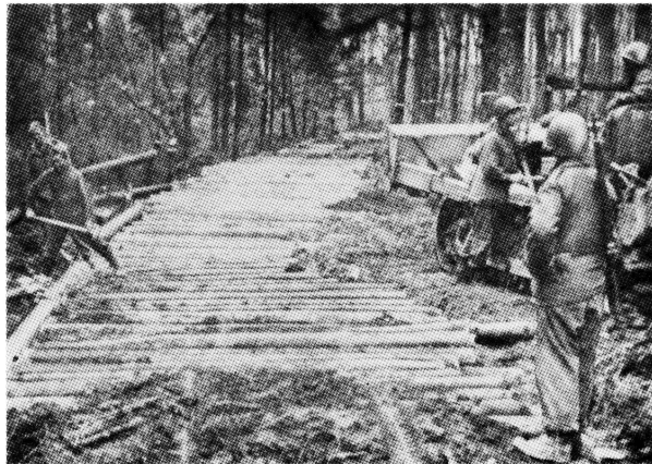
b. Corduroy road being covered with an earth wearing surface.
