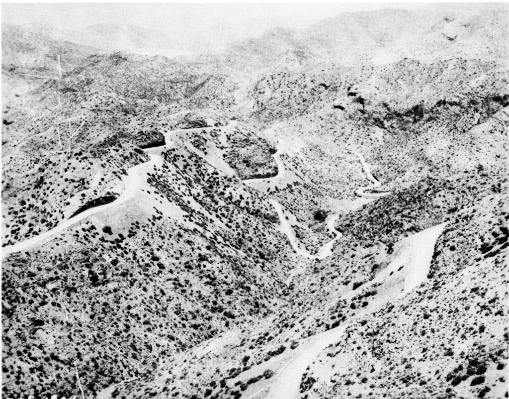
Figure 17. Road with steep grades and sharp curves.
