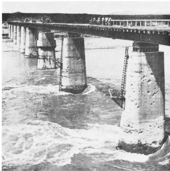
Figure 28. Solid concrete pier.
