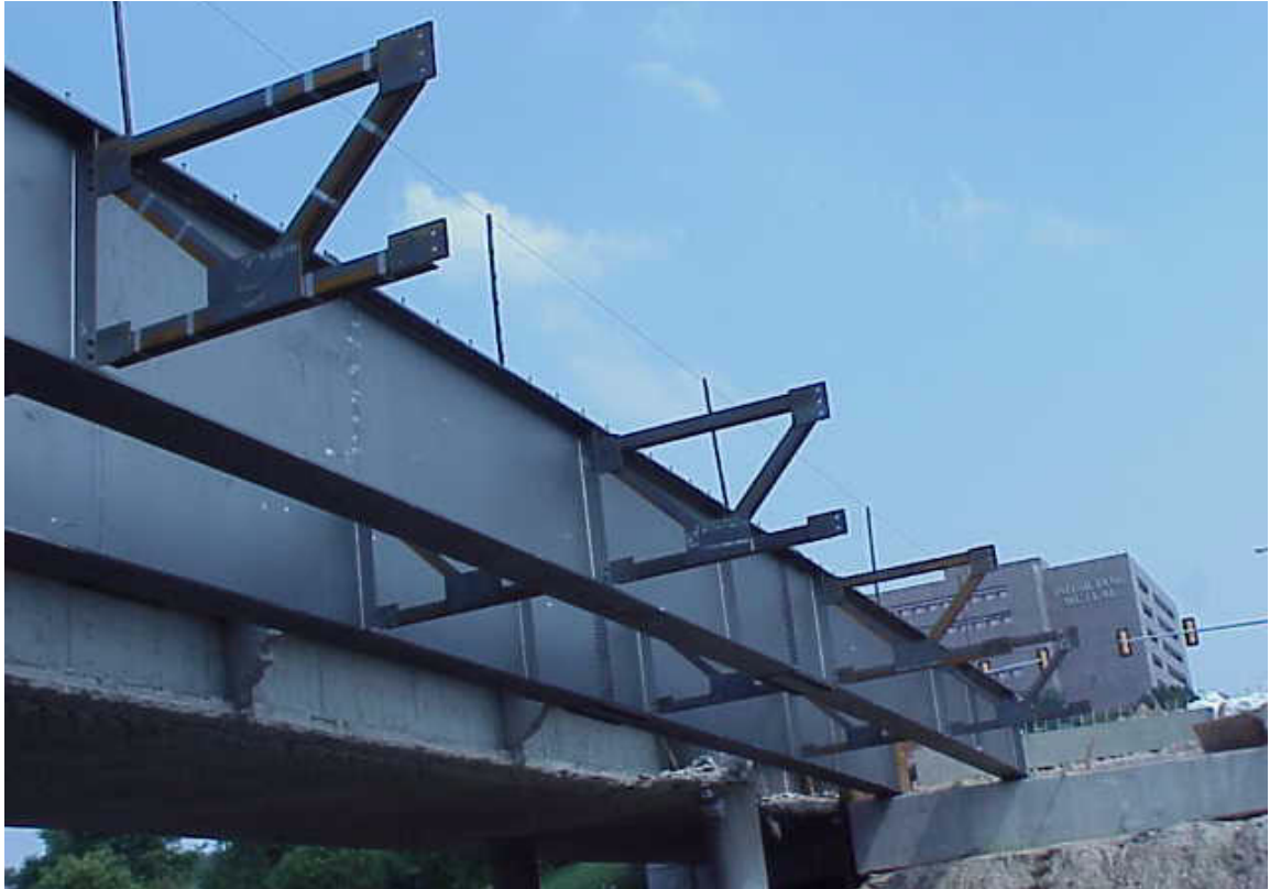
Figure 2-11: Girder sections 4 and 5 of the East span
