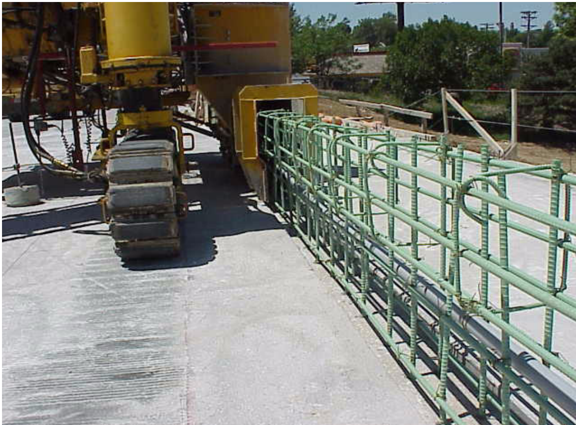
Figure 2-28: Phase II permanent barrier before casting. Note dowels epoxied into deck
