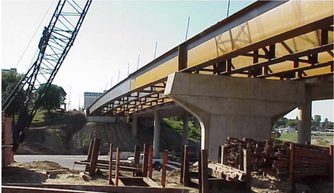
Figure 2-13: West span girders in place
