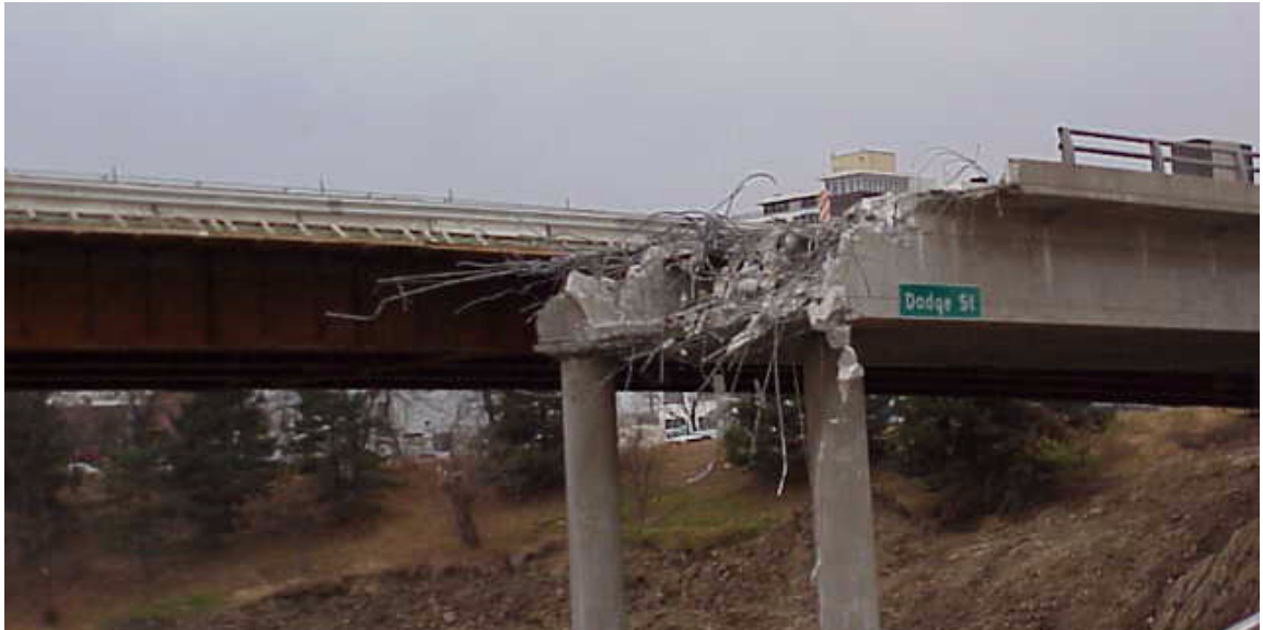
Figure 2-18: Demolition of the Northern half of the existing bridge
