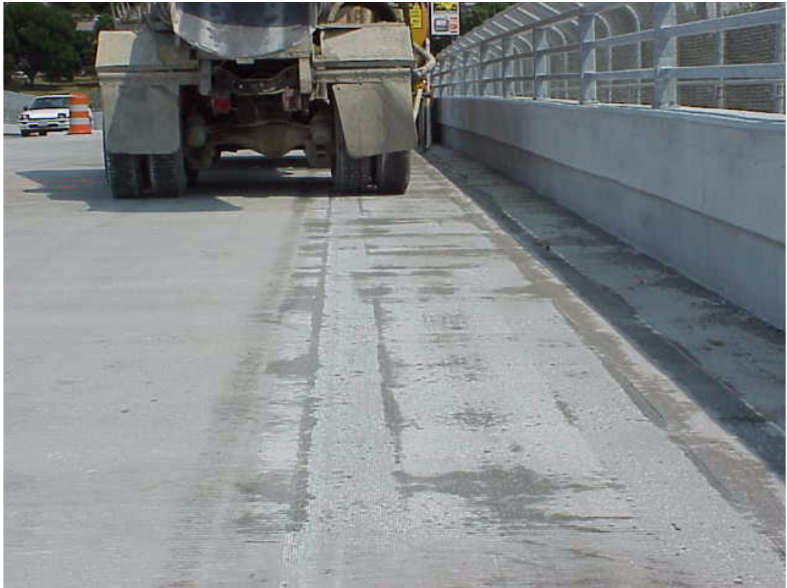
Figure 2-31: Finished permanent barrier. Note truck on bridge is grinding surface.
