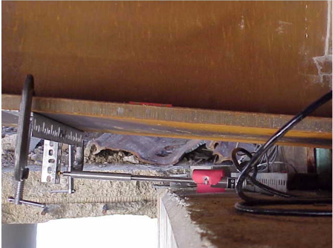
Figure 2-37: Crackmeter connected to girder flange
