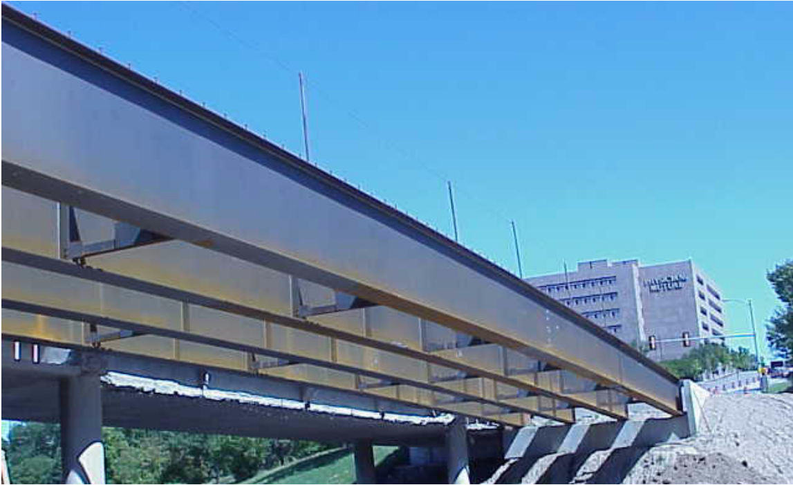
Figure 2-12: All four girders for East span in place.
