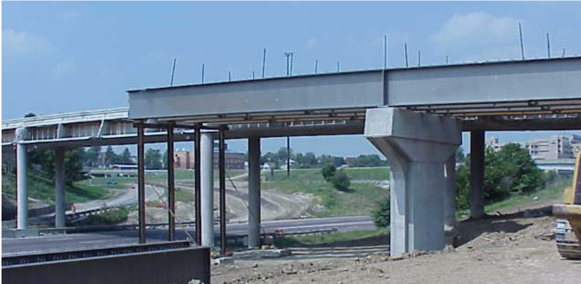
Figure 2-10: Girder sections E3, G3, H3, and J3 placed over the pier
