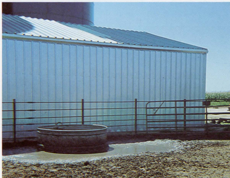
Fig. 12.—Water tank runoff
