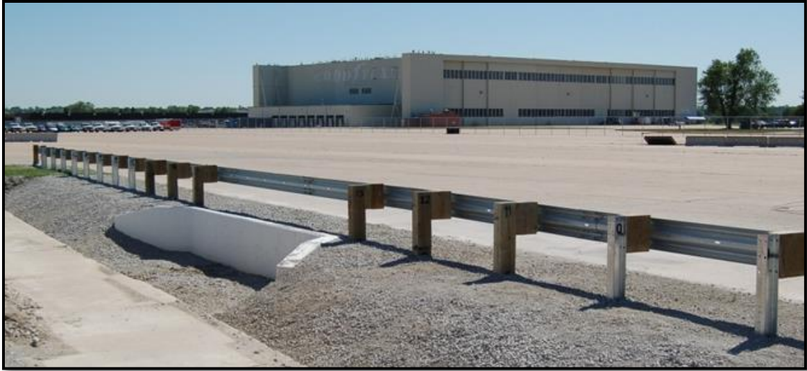
Figure 1. Midwest Guardrail System 25-ft Long-Span Design
