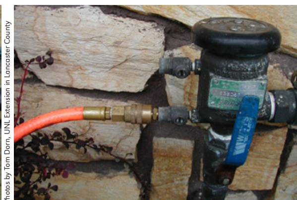
To let air into lawn sprinkler systems, open the small valves (petcocks) on the vacuum relief valve assembly (shown at left), or to be extra safe, attach an air compressor to the lower petcock valve (shown at right).
