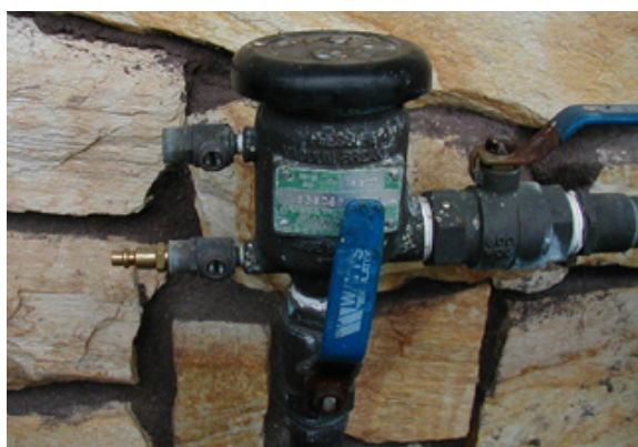
To let air into lawn sprinkler systems, open the small valves (petcocks) on the vacuum relief valve assembly (shown at left), or to be extra safe, attach an air compressor to the lower petcock valve (shown at right).
