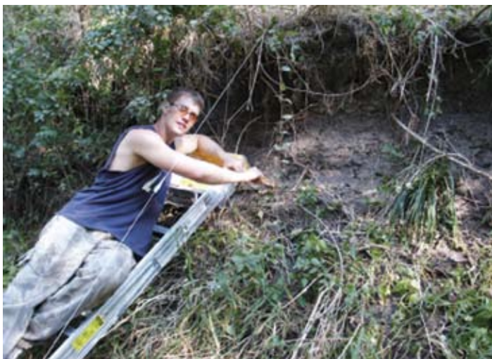
Above: Nathan installing small welding rods or pins in stream banks.
