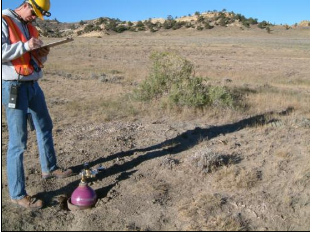
Site 2C – Underground leak located in gravel area approximately 8 feet from bottle location.
