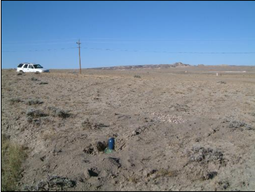
Site 2E – Underground leak located in the gravel area approximately 8 feet from bottle location. Vehicle located on the road.
