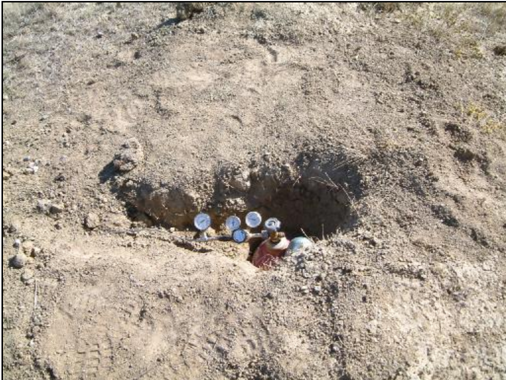
Site 2A – View of bottle and regulator (typical of all bottle fed leaks; 2A through 2E).
