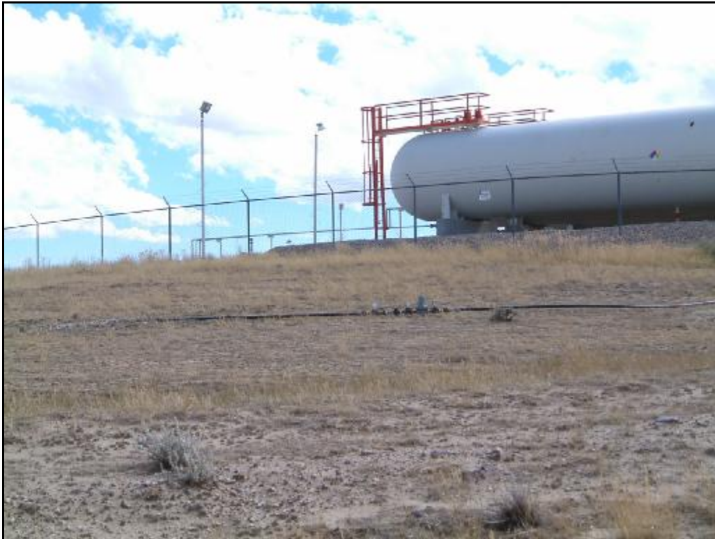
Site 5 – View from the road.
