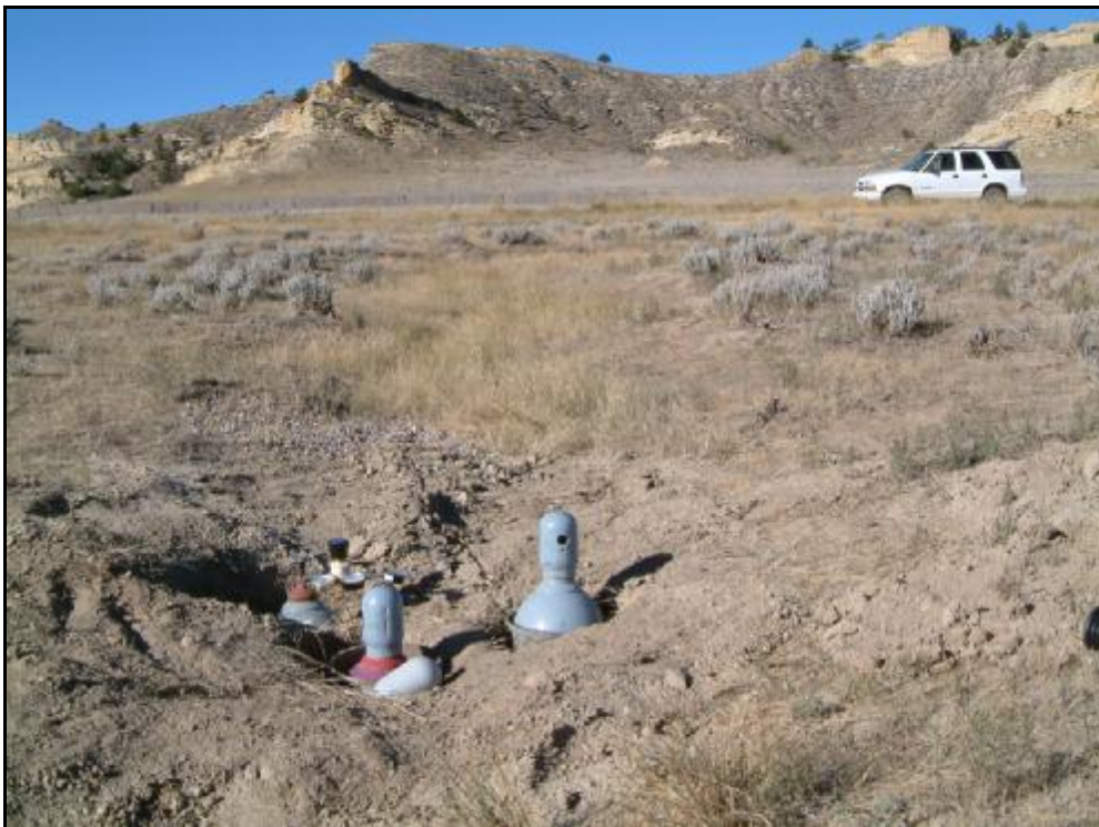
Site 2D/Site 1F – Three bottles (two with methane only, one with methane/ethane mix). Underground leak located in the gravel area approximately 8 feet from bottle location. Vehicle located on the road.
