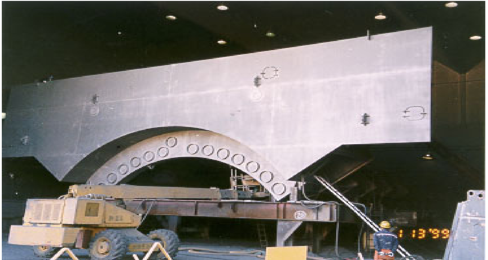
Block after removal of PCP
