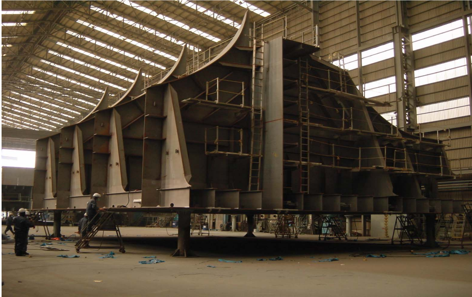
Block Assembly in Fabrication Hall
