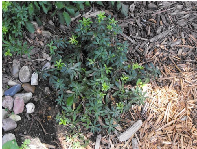
(Fig. 7) Clogged rock overflow showing encroaching mulch needing redistribution.
