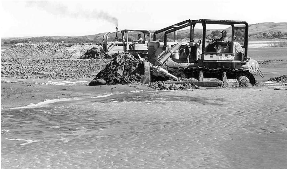
Figure 3 Dozers Constructing ESH
