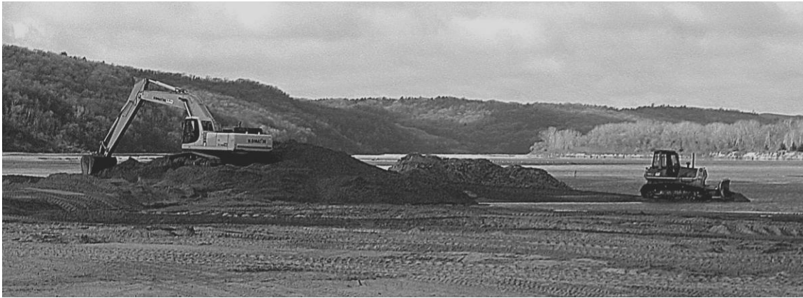
Figure 1 Excavation for Emergent Sandbar at River Mile 761.3
