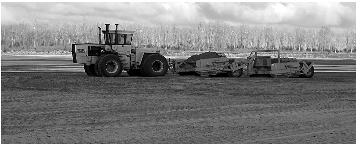
Figure 2 Pan Scrapers Constructing ESH
