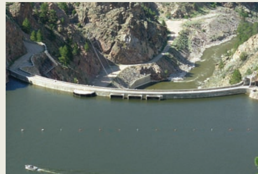
After years of unprecedented drought, reservoirs in the U.S. Bureau of Reclamation's North Platte Project in Wyoming are at or nearing capacity. Shown here in Seminole Dam and Reservoir.
