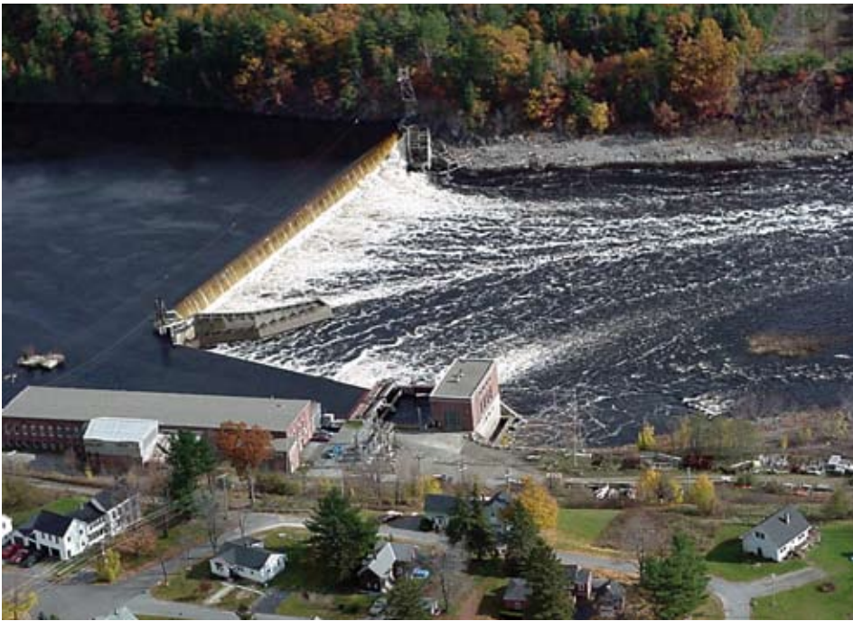
Veazie Dam, one of the dams to be removed to enhance fish passage.
