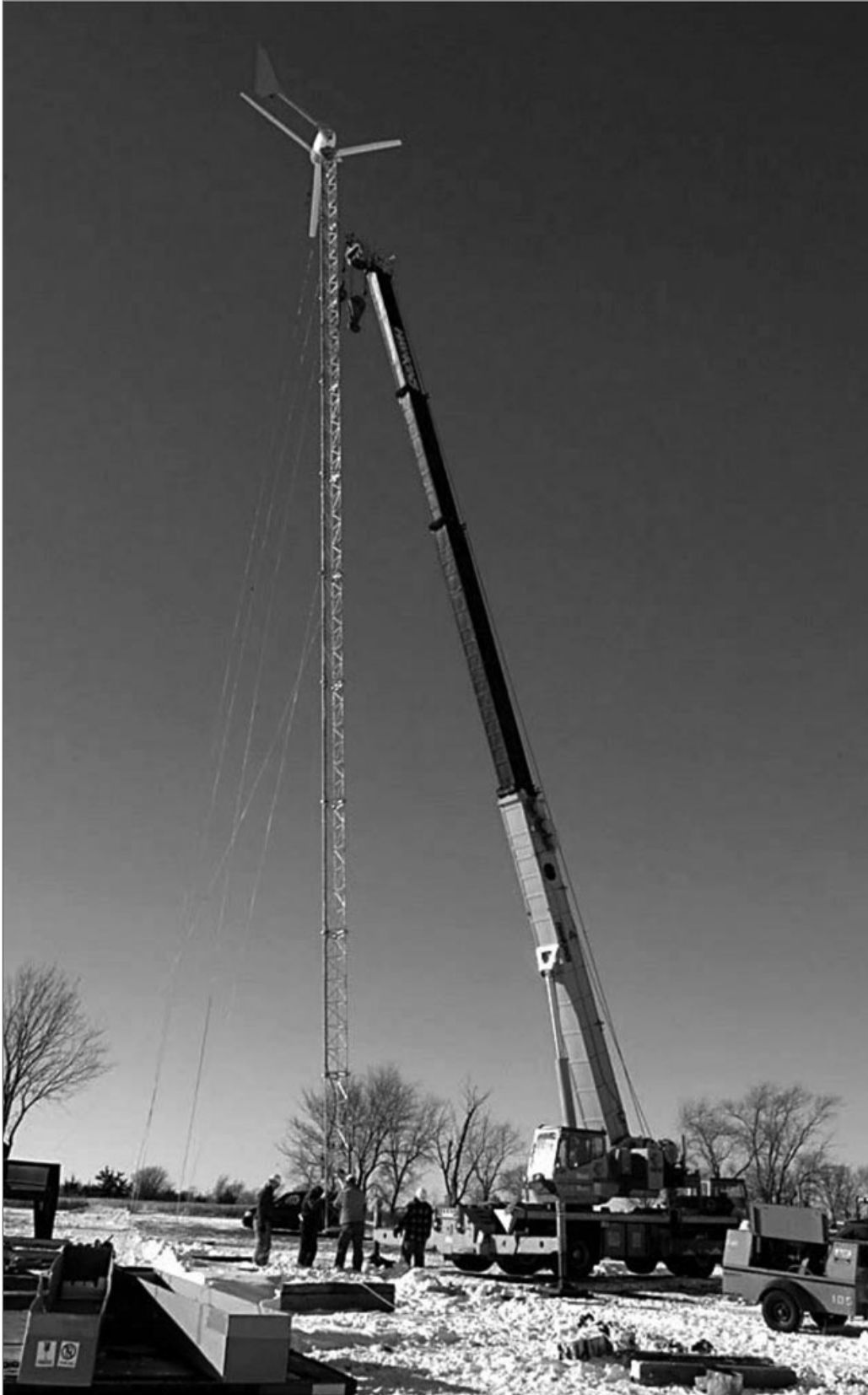
Exhibit 3. Erection of the wind turbine in December 2003
